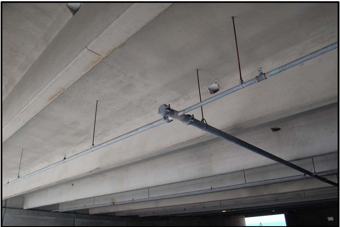
PRE-STRESSED CONCRETE STRUCTURAL FEATURES AND FIRE SPLINKLER
