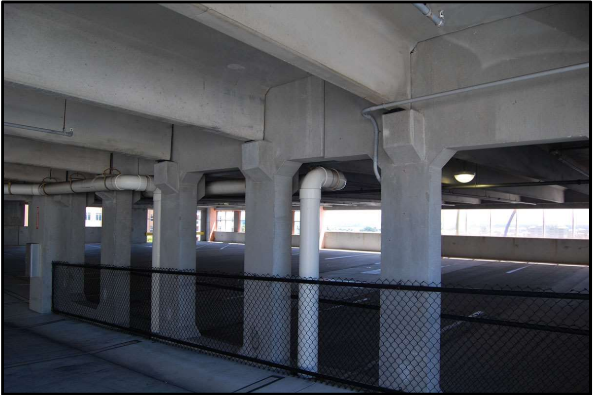
PVC ROOF DRAINS AT 6 TH LEVEL
