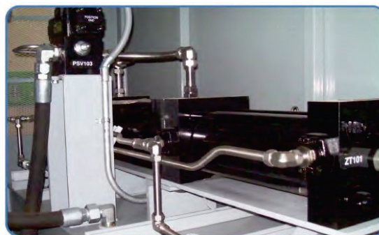
Hy-C compressor installed at a public fueling station
