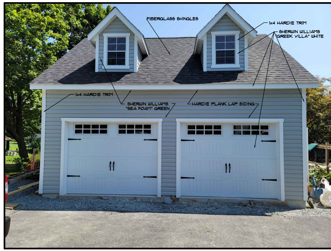
SIDING, TRIM & ROOFING MATERIAL & COLOR 2ND LEVEL NO SCALE
