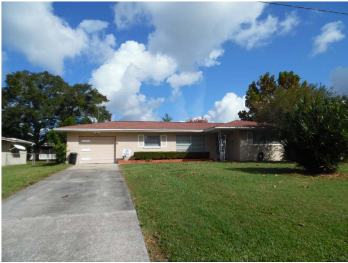
View looking north at the subject property, 2140 Burnice Drive
