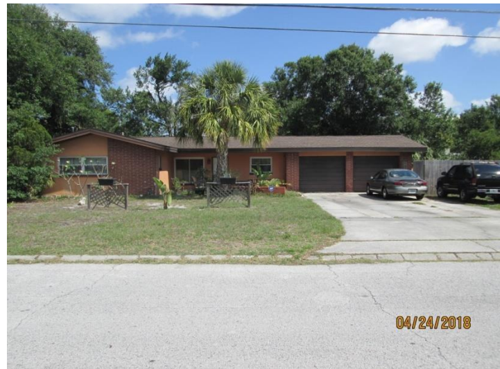
View east of the subject property, along Barry Road
