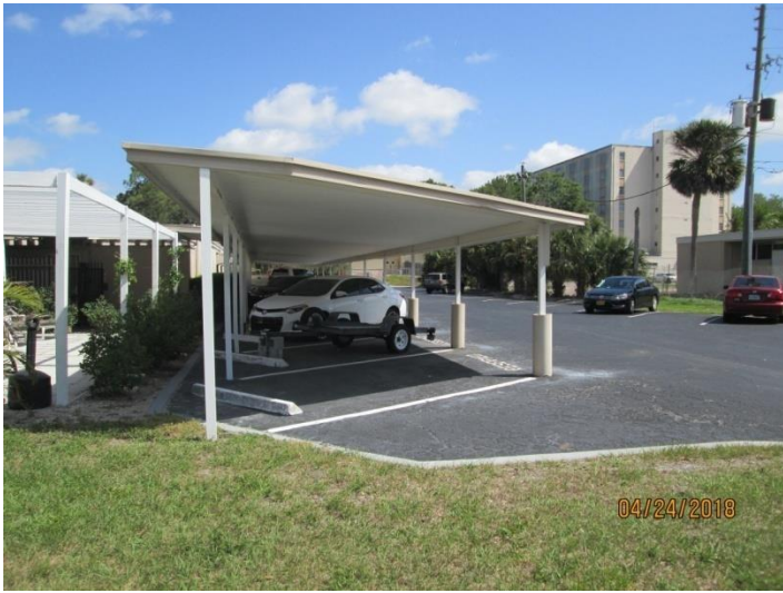
View west of the subject property, along Barry Road
