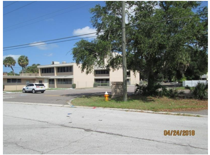
View looking north at the southeast corner of the subject property, from Barry Road.
