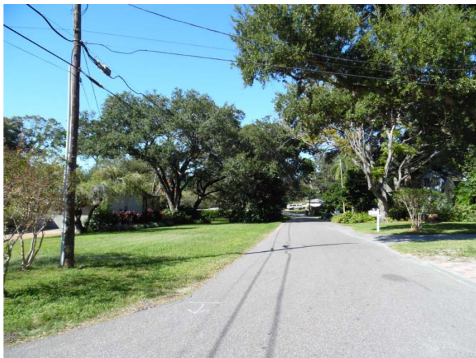
Looking westerly along Bell Cheer Drive
