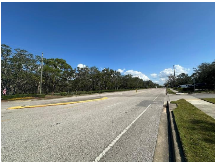
Facing east along Sunset Point Road
