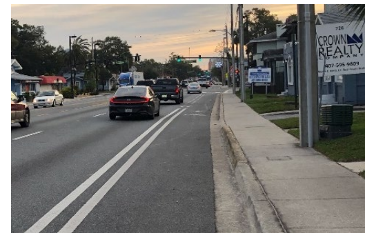
Image 8: Painted Buffered Bike Lane
