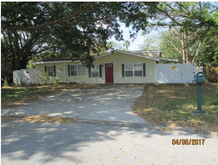
South of the subject property
