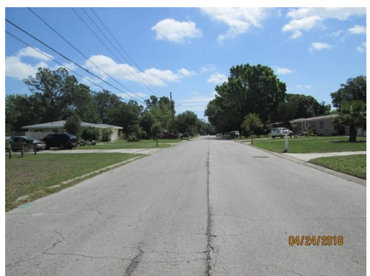
View looking easterly along Barry Road, along the southern property line of the subject property
