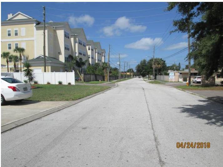
View looking westerly along Barry Road, along the southern property line of the subject property
