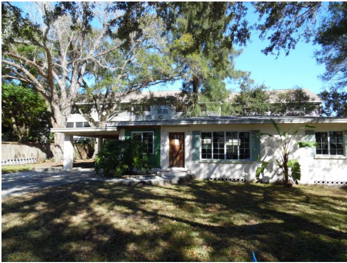
View looking north at the subject property, 3128 Johns Parkway
