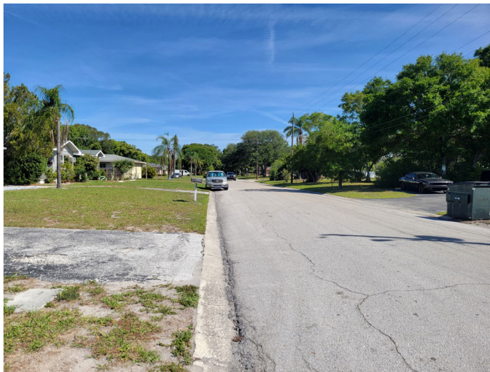
View looking northerly along S Mars Avenue
