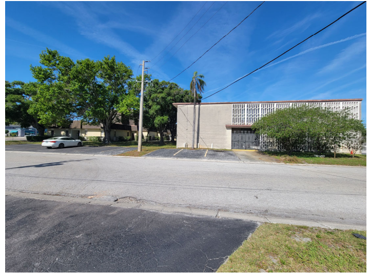
View looking west at the subject property
