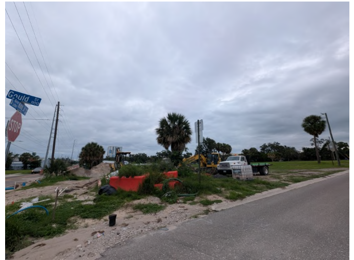
View Looking Northeast Across Subject
