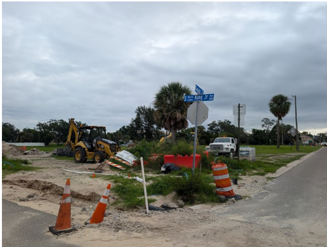
View Looking Northeast Across Subject
