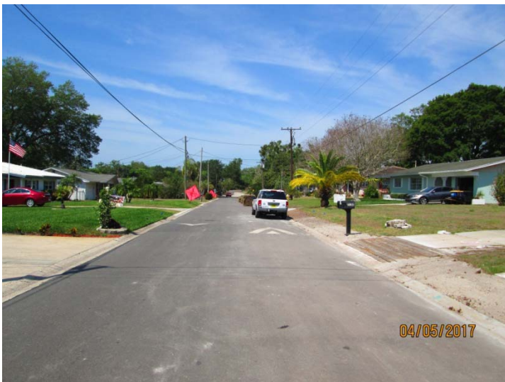
View looking westerly along Burnice Drive
