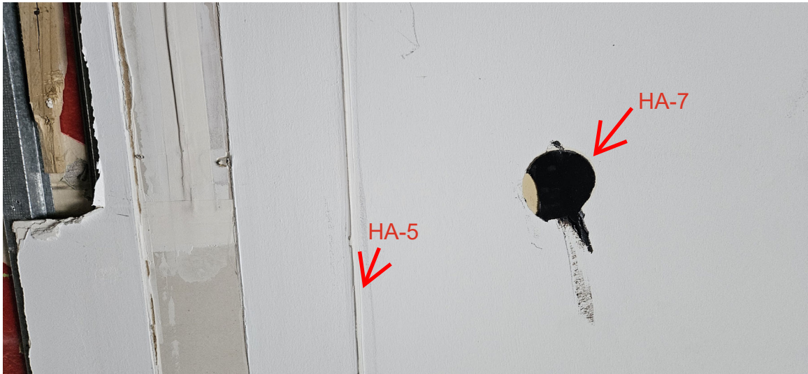
Homogeneous Area #5: White Caulking Homogeneous Area #7: Black Mirror Mastic
