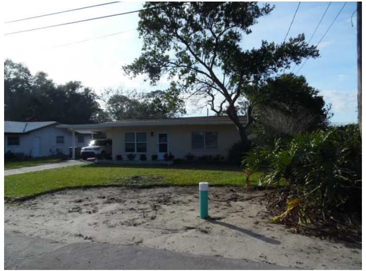
Across the street, south of the subject property
