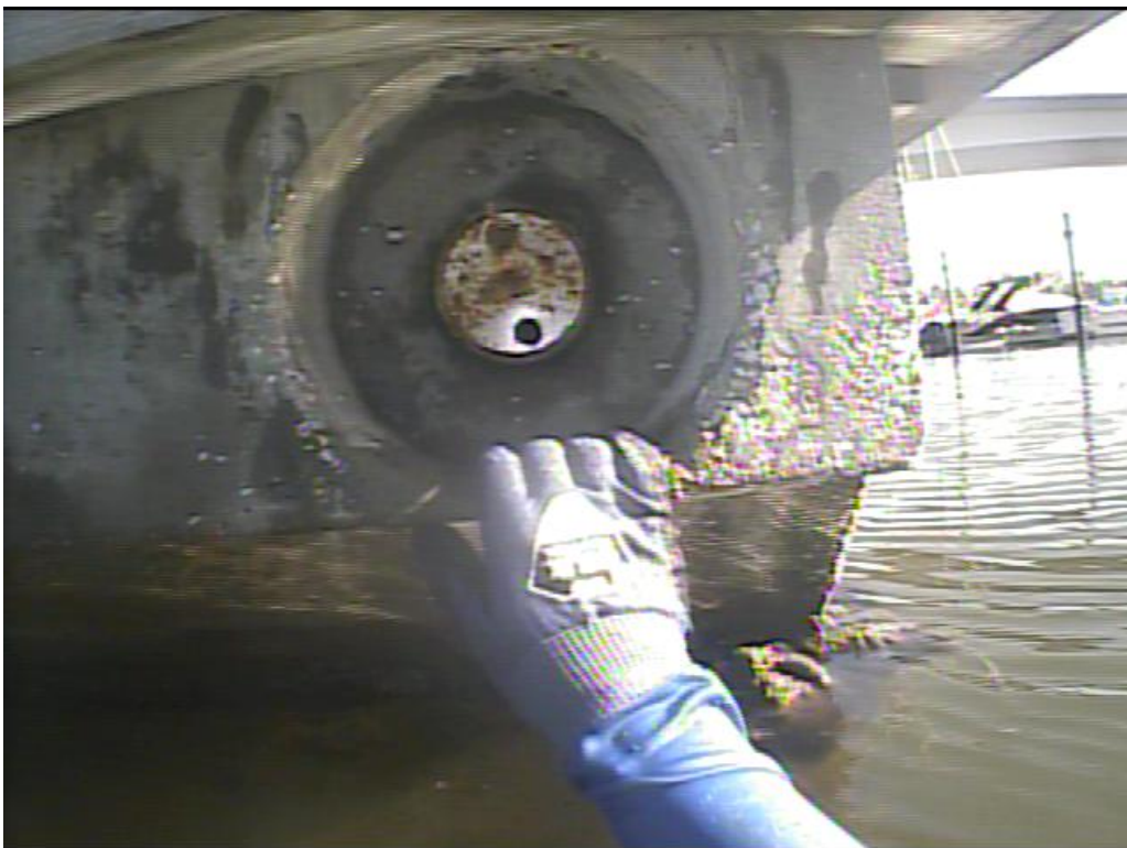
Photo 7: Concrete Spalling around Cable Sleeve
