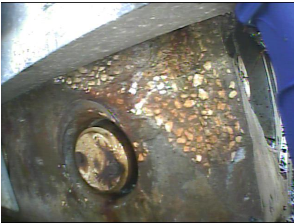
Photo 11: NW Corner Concrete Spalling
