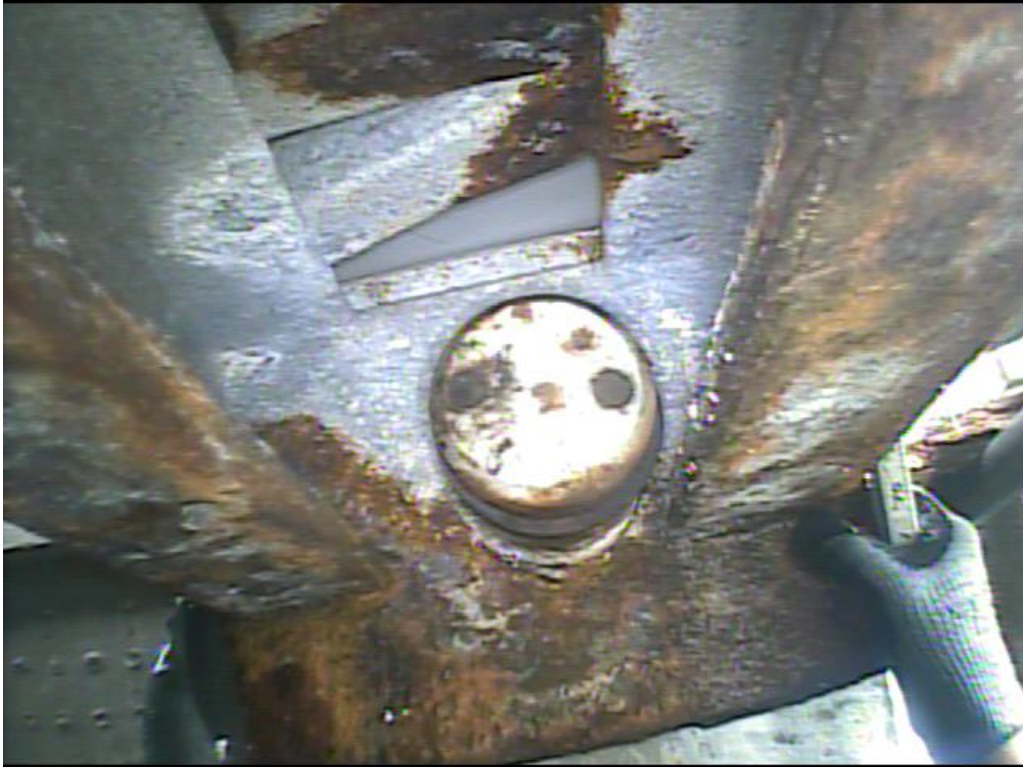
Photo 18: Corroded Cable End
