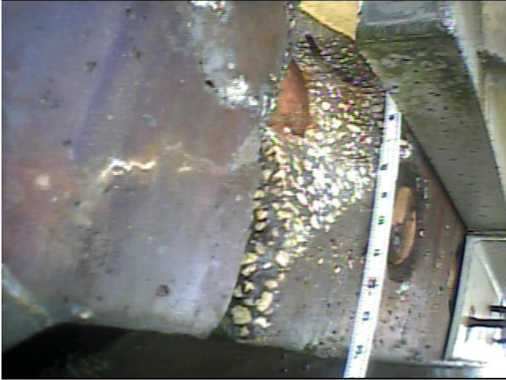
Photo 12: NE Corner Exposed Steel Conduit for Cable
