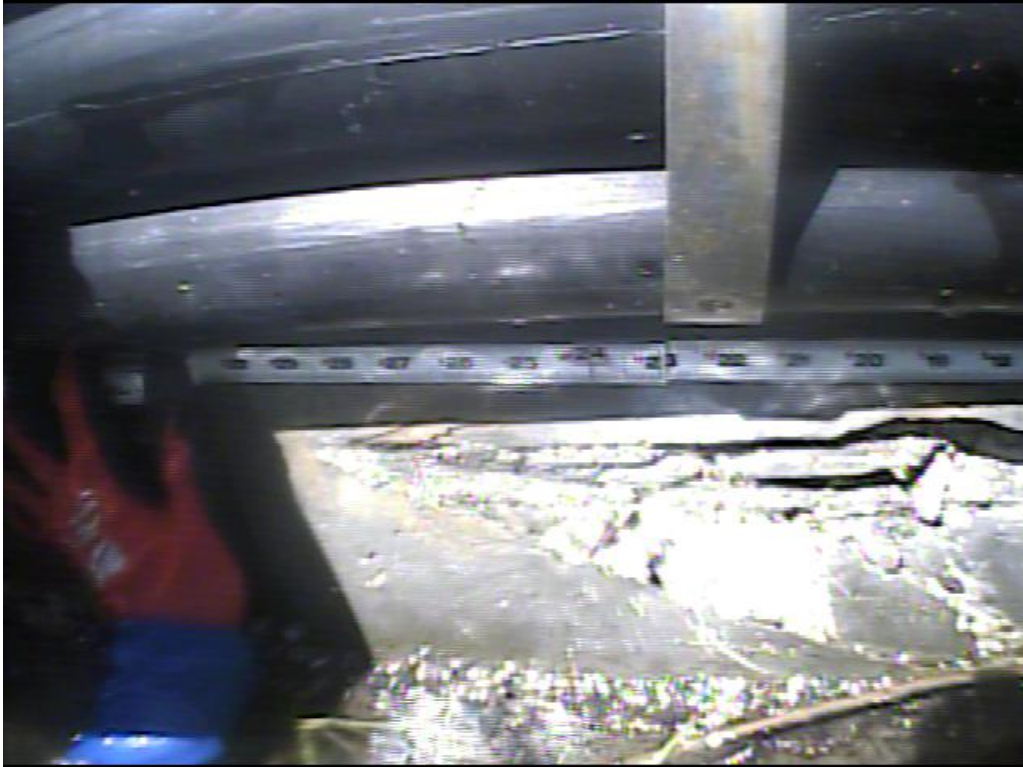
Photo 4: Large Concrete spall
