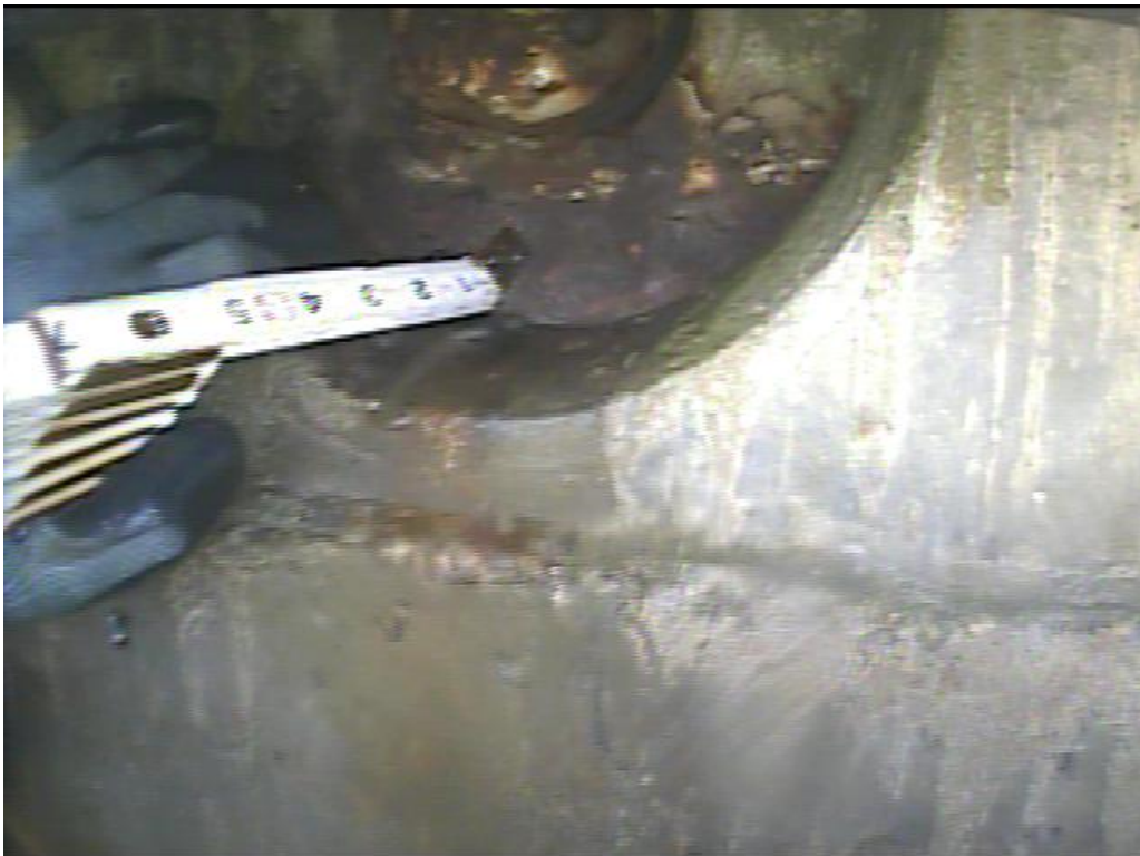
Photo 2: Cable Corrosion Around Cable End
