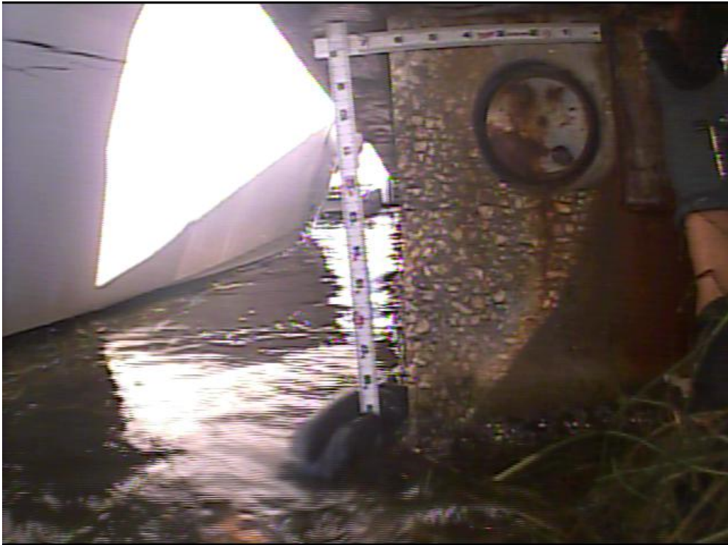
Photo 14: NW Corner Concrete Spalling
