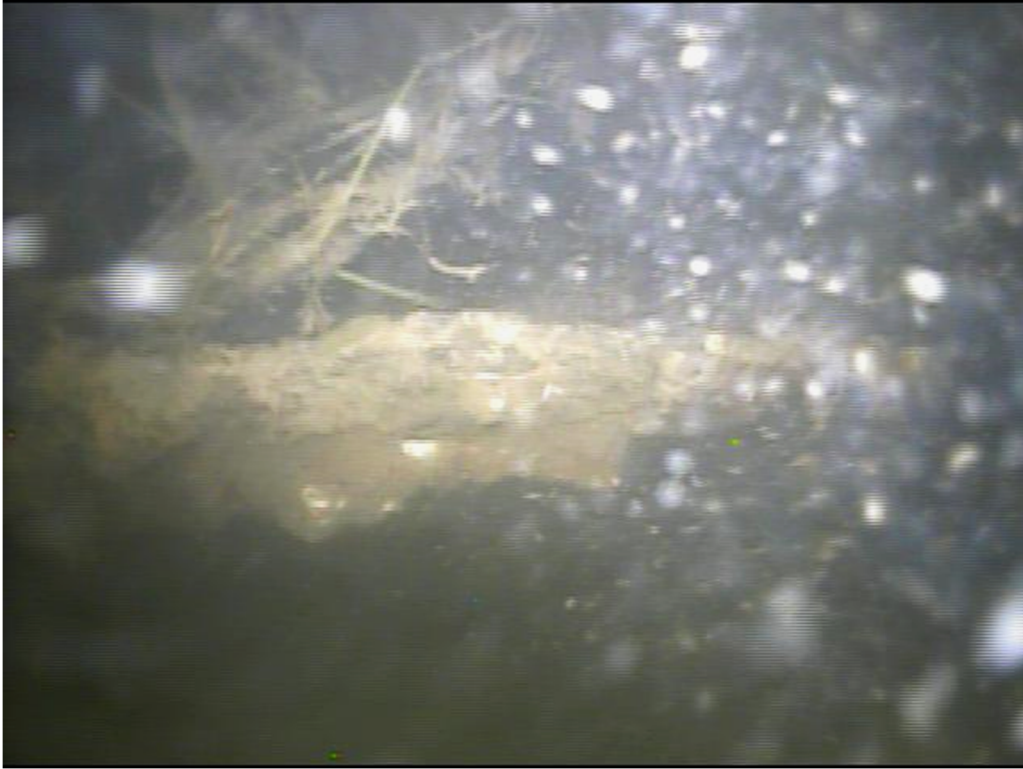
Photo 1: Polyurethane Liner Tear and Exposed Foam
