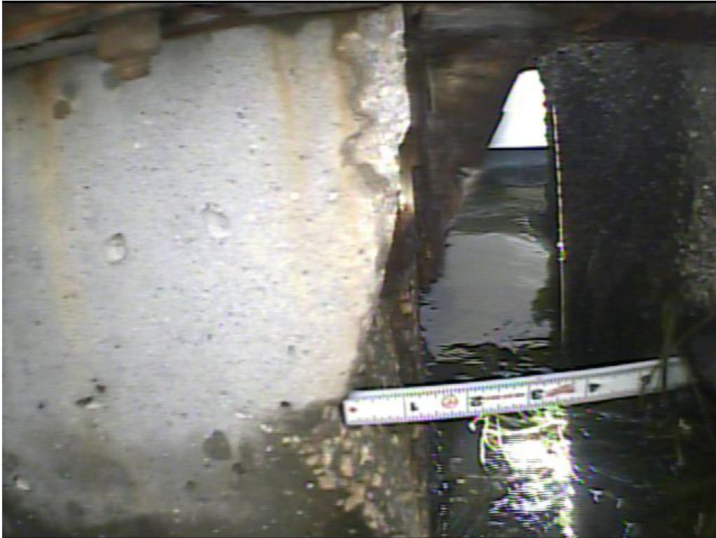
Photo 13: NW Corner Spall
