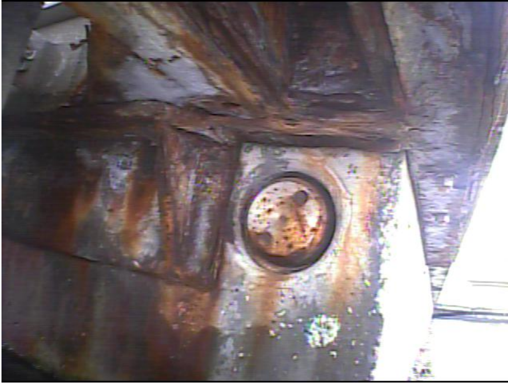
Photo 16: Corroded Cable End
