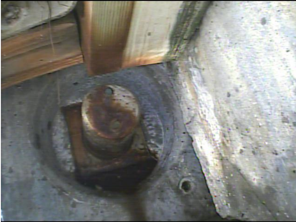
Photo 9: Cable Corrosion
