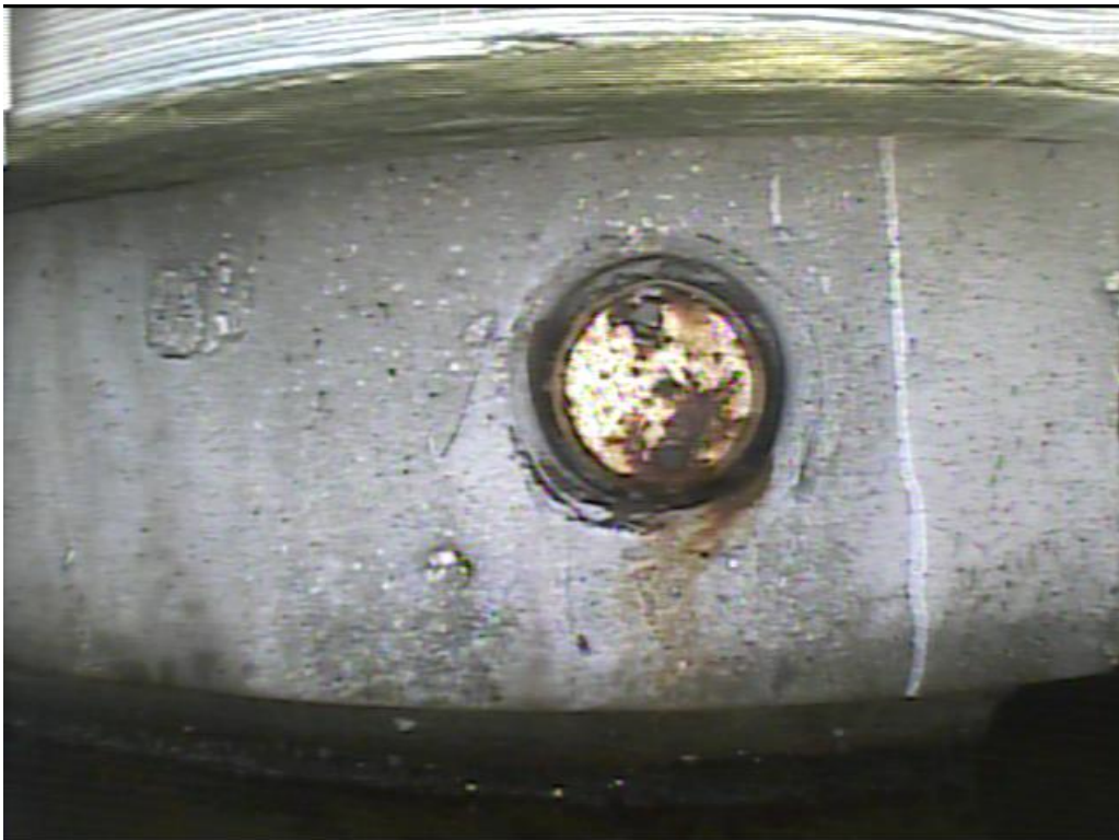
Photo 5: More than Average Cable Corrosion
