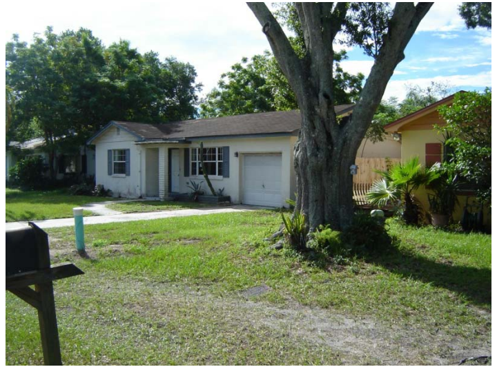
East of the subject property
