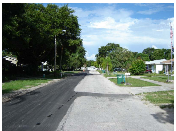
View looking westerly along Palm Street
