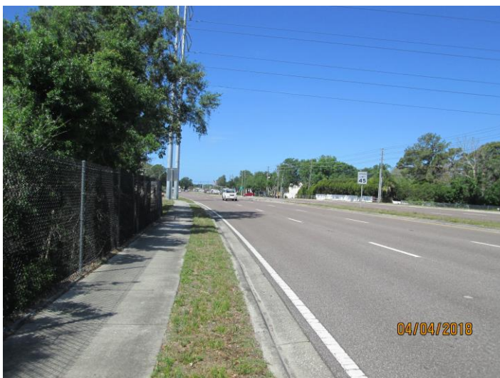
View looking westerly along Curlew Road
