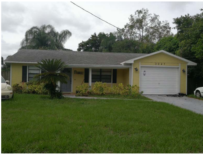
View looking south at subject property, 3047 Lake Vista Drive
