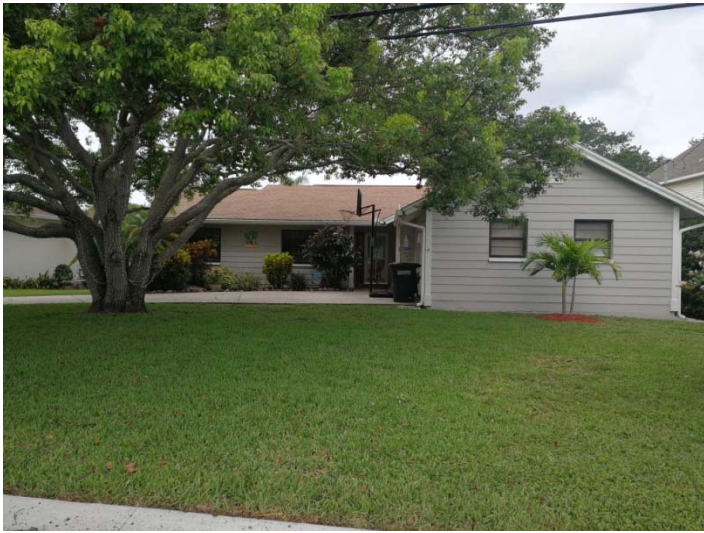
View looking west at subject property, 712 Moss Avenue
