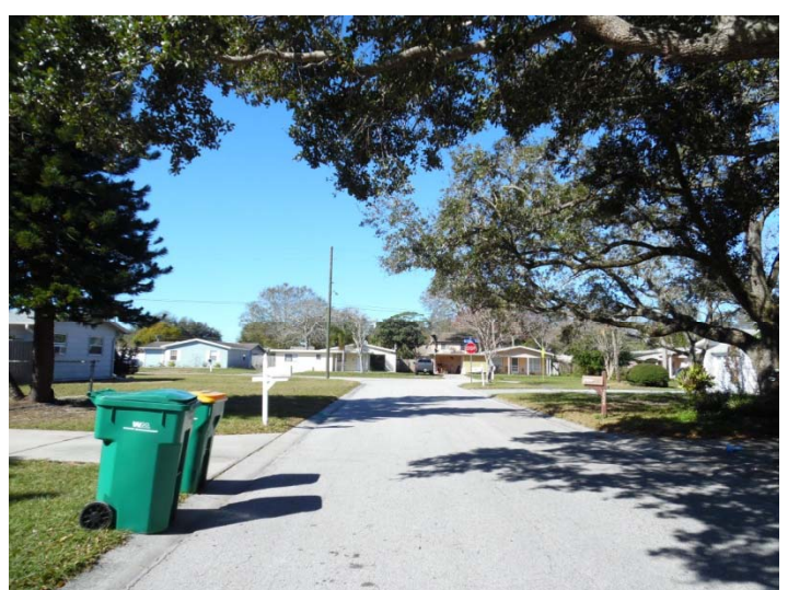
View looking westerly along St. John Drive
