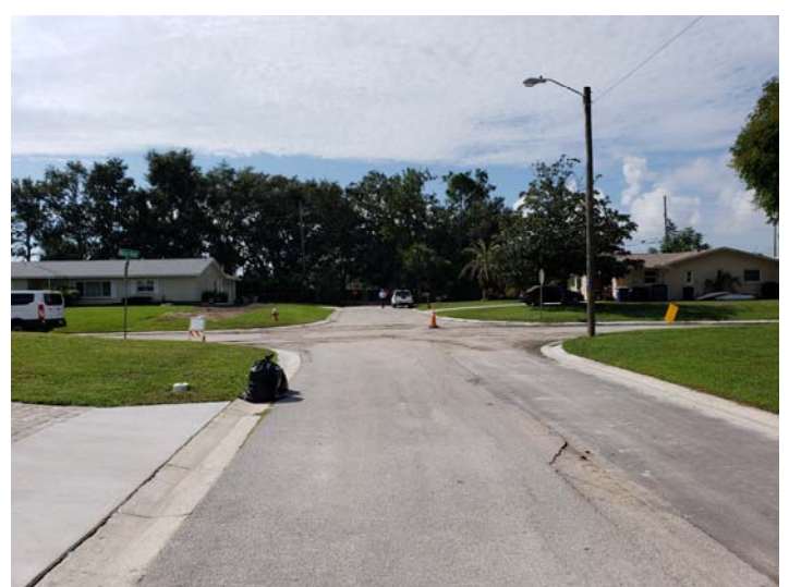
View looking southerly along Moss Avenue
