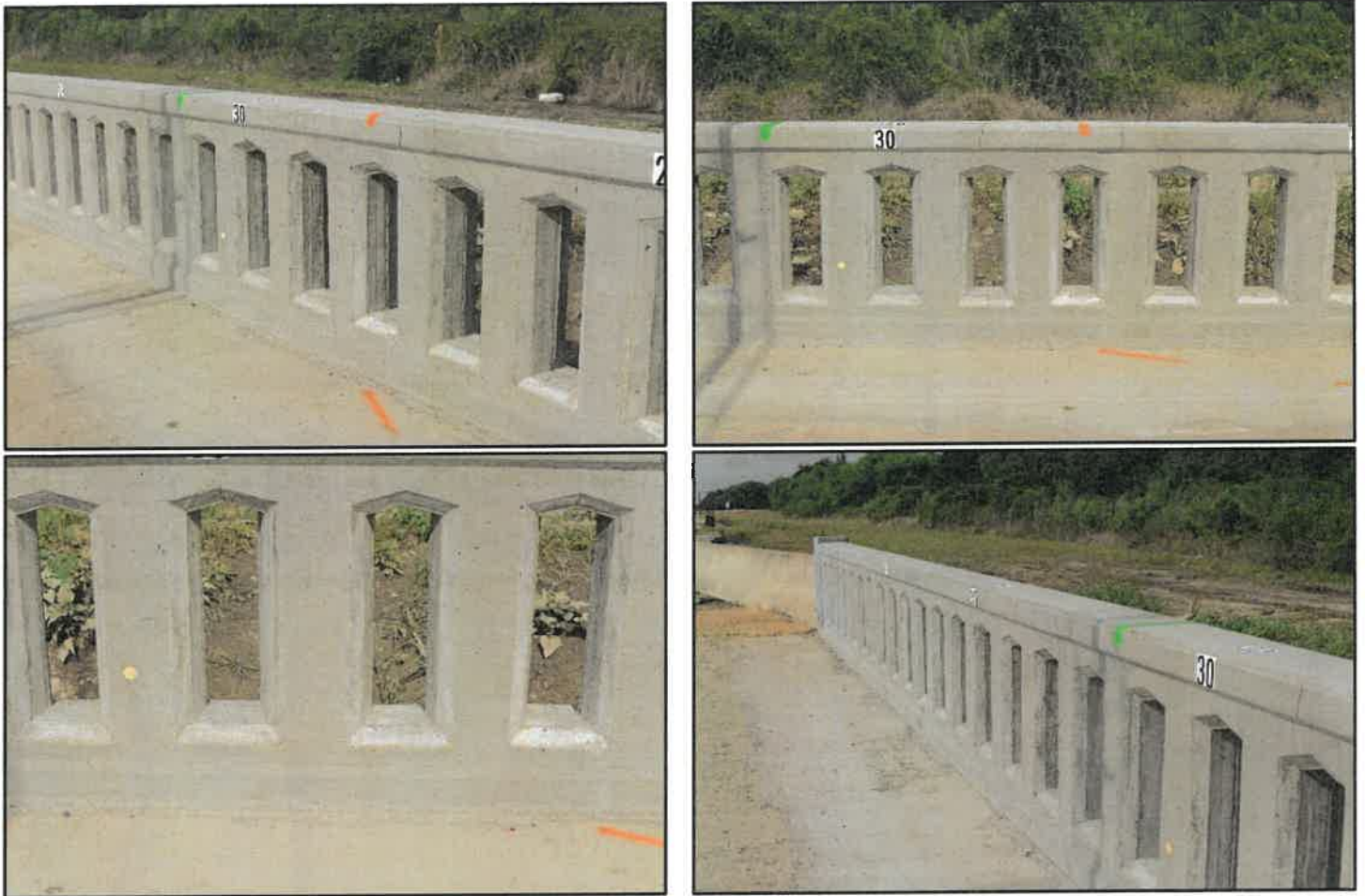
Figure 4.2. TxDOT C411 Bridge Rail prior to Testing.
