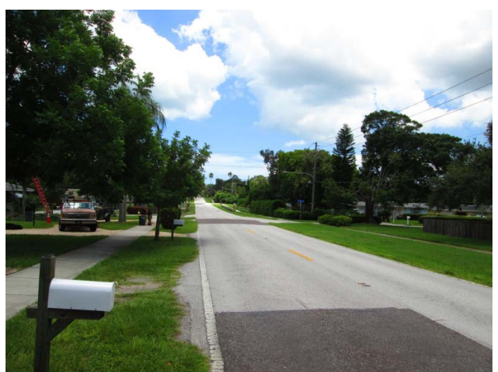
View looking westerly along Lakeview Road
