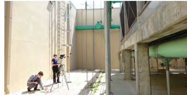
Figure 9. Acoustical measurements and recordings taken of the air intake sides of the cooling towers at an existing facility similar to the proposed central energy plant.
