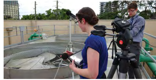
Figure 8. Acoustical measurements and recordings of the cooling tower fans taken at an existing facility similar to the proposed central energy plant.
