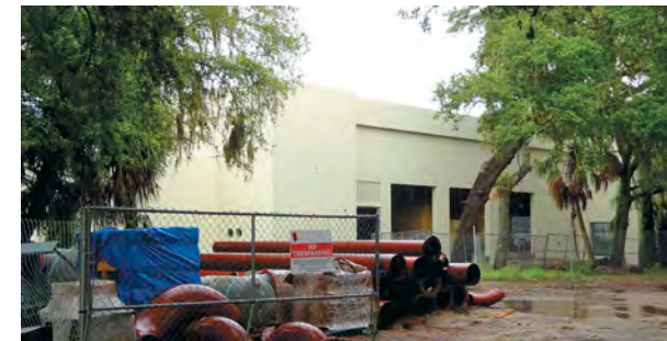
Figure 16. Acoustical measurements will be taken once construction is complete to verify the sound levels measured during the simulation. This image shows the chiller building before doors are installed and chilled water pipes stored on site.
