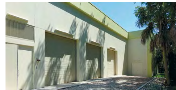
Figure 17. Acoustical measurements will be taken once construction is complete to verify the sound levels measured during the simulation. This image shows the installation of doors and roll-up doors in the chiller building. The man door to the right of the image opens into the cooling tower well.
