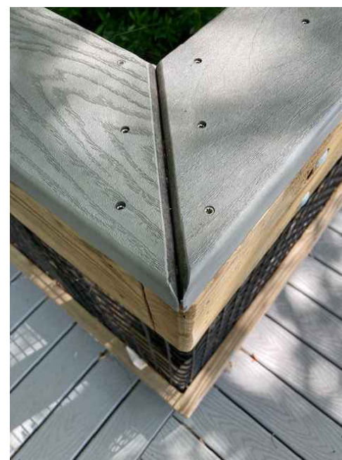
DETAIL C MITERED CORNER W/ BEVEL EDGES
