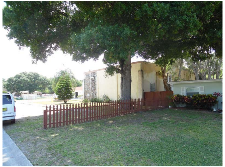
East of the subject property
