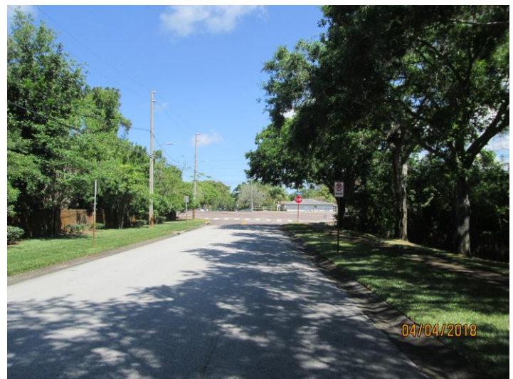
View looking northerly along Lake Shore Lane
