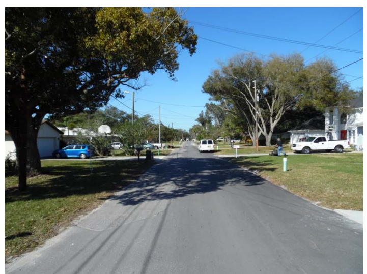
View looking westerly along Bell Cheer Drive
