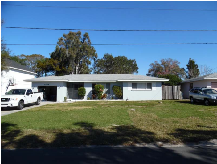
View looking north at the subject property, 2174 Bell Cheer Drive
