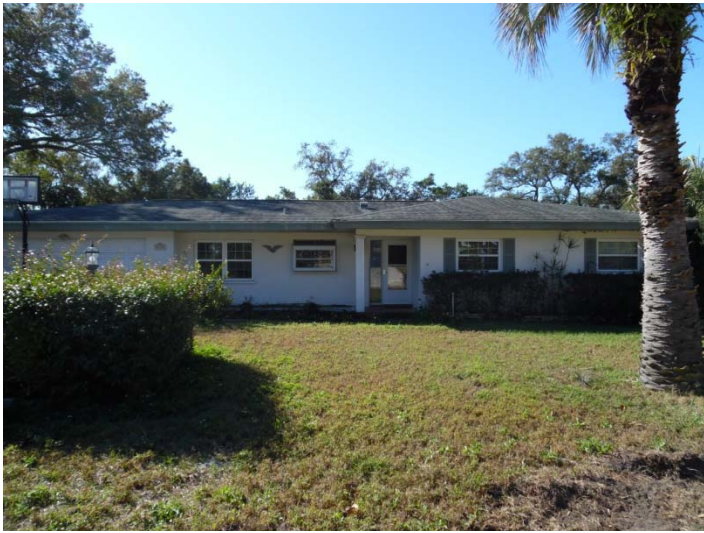
View looking south at the subject property, 2109 Burnice Drive
