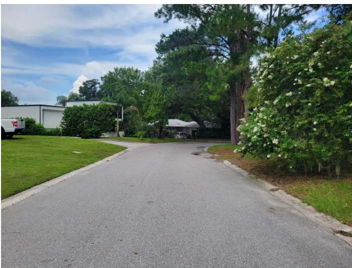
View looking westerly along Pleasant Parkway
