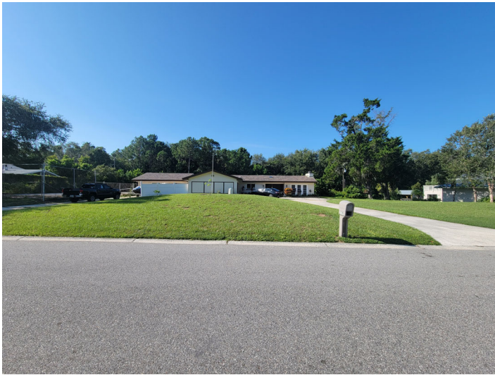
View looking south at subject property 2135 Pleasant Parkway
