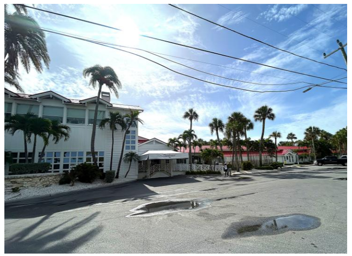
Facing east from Eldorado Avenue towards clubhouse and pool building (right)
