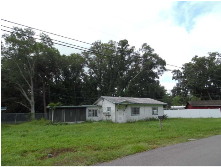
View looking east at the subject property, 2727 Daniel Street
