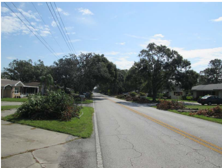
View looking easterly along Lakeview Road
