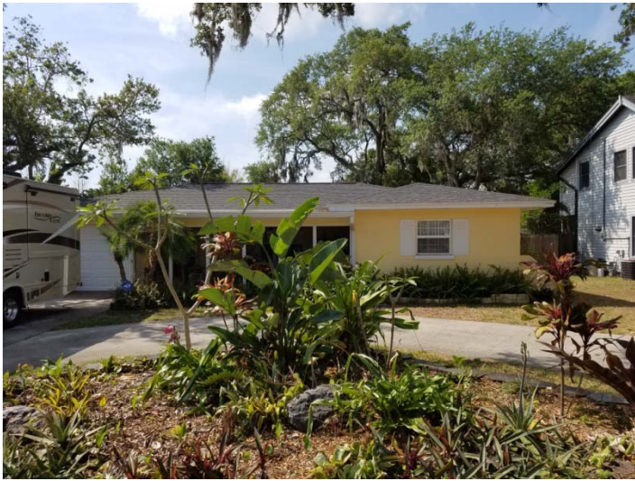
View looking south at the subject property, 3121 Wolfe Road
