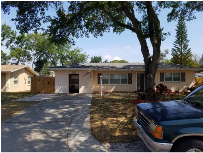
View looking north at the subject property, 3064 Grand View Avenue
