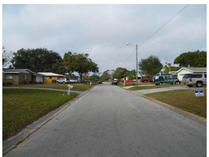
View looking westerly along Hoyt Avenue
