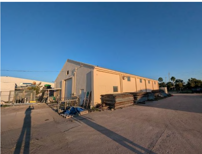
View of Electric Service
