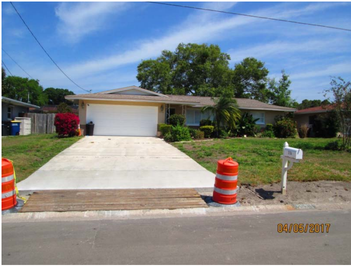
View looking north at the subject property, 2134 Burnice Drive
