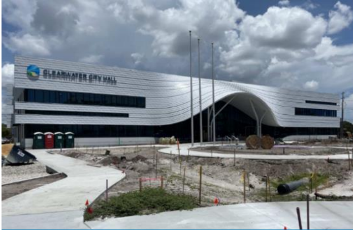
City Hall Construction
