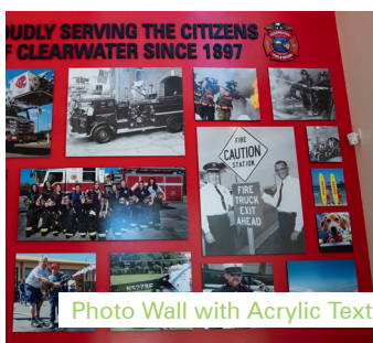
Acrylic Wall Installation
