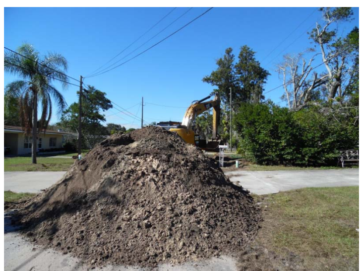
View looking westerly along Bell Cheer Drive
