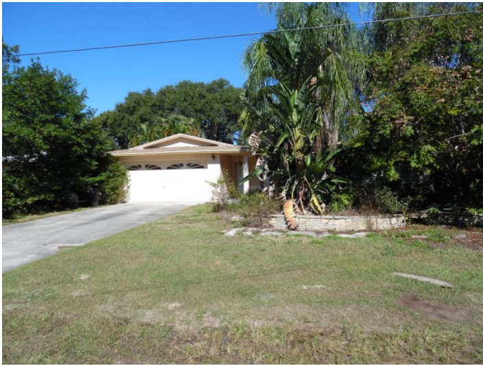
View looking north at the subject property, 2142 Bell Cheer Drive
