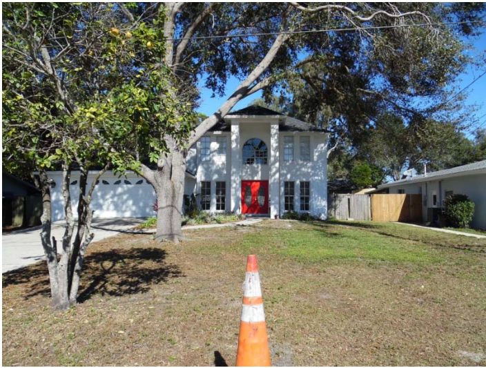
View looking north at the subject property, 2166 Bell Cheer Drive
