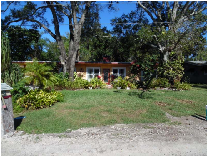
View looking north at the subject property, 2118 Bell Cheer Drive
