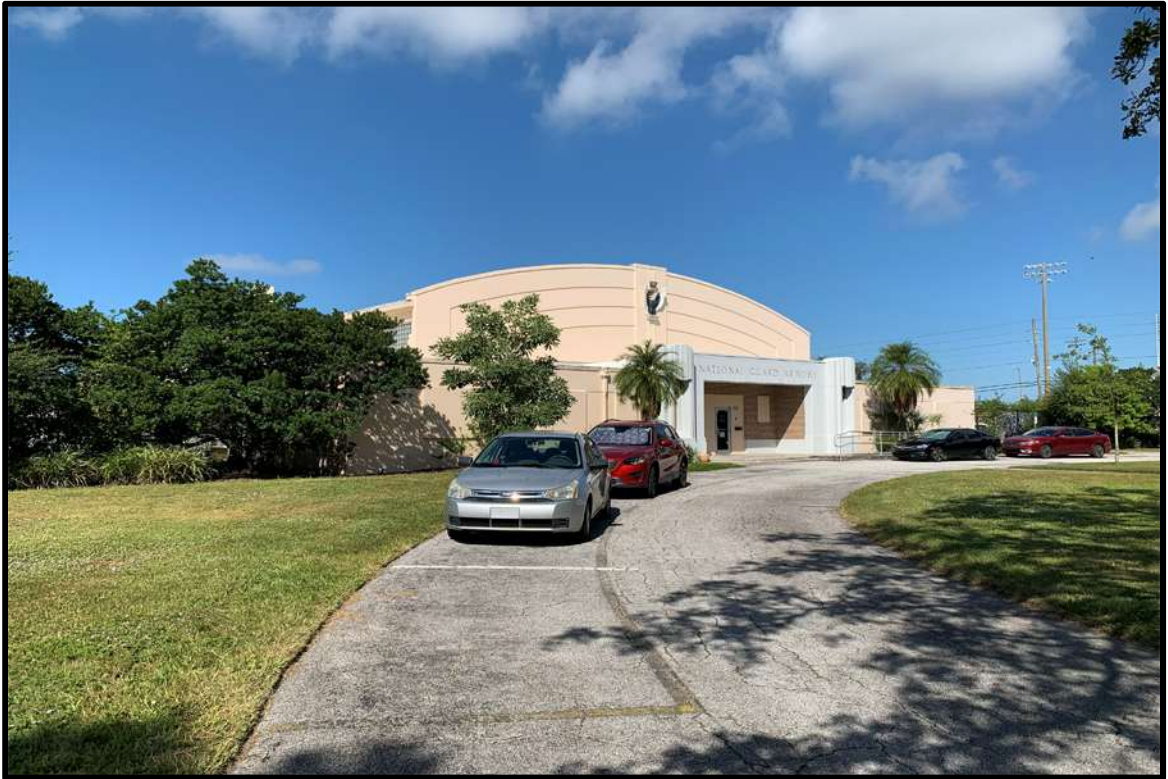
FRONT VIEW OF ARMORY (BUILDING A) FROM SOUTHEAST
