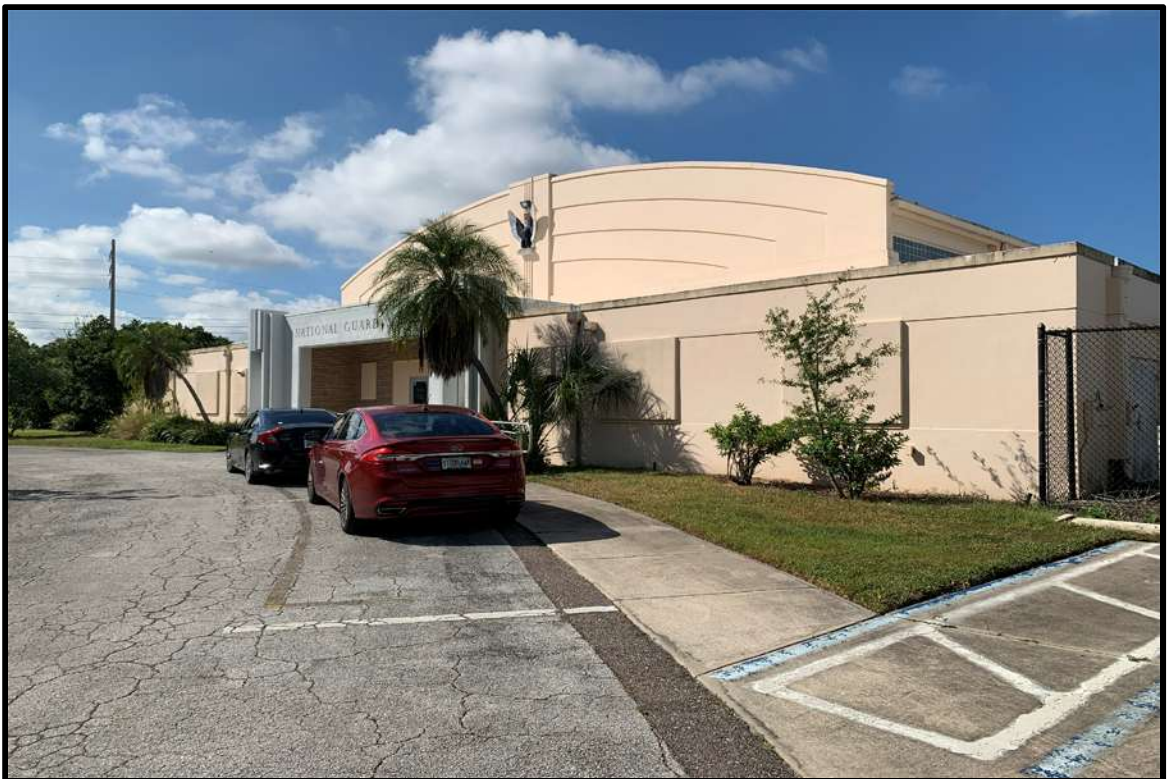
DETAIL FRONT VIEW OF BUILDING A FROM NORTHEAST
