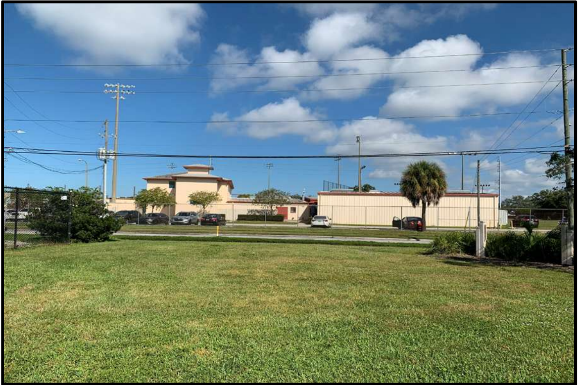
JACK RUSSELL STADIUM; VIEW NORTH FROM SUBJECT
