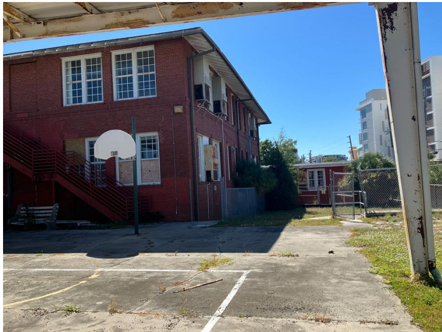
BACK BUILDING VIEW LOOKING TOWARD KITCHEN
