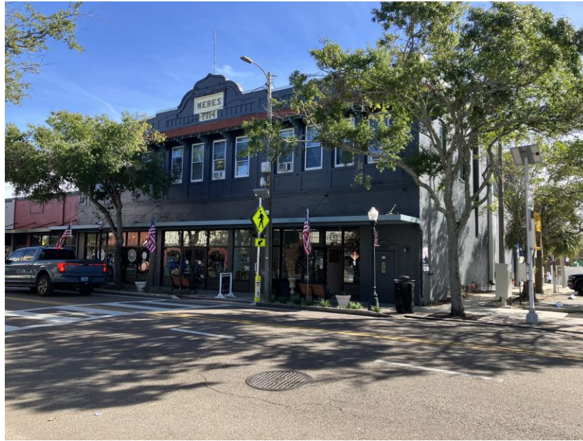
MERES BUILDING (1914) 106 E. TARPON AVENUE, TARPON SPRINGS NOVEMBER 5, 2025
