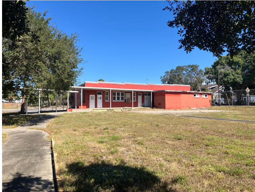
BACK VIEW OF ANNEX BUILDING SCHOOL YARD
