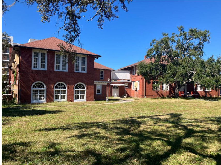
MAIN BUILDING VIEW FROM N. FT. HARRISON AVENUE
