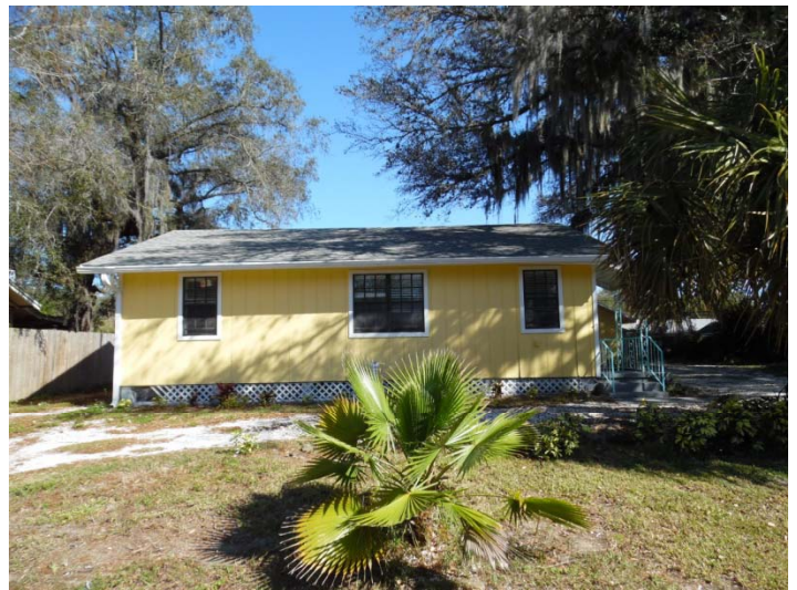
West of the subject property
