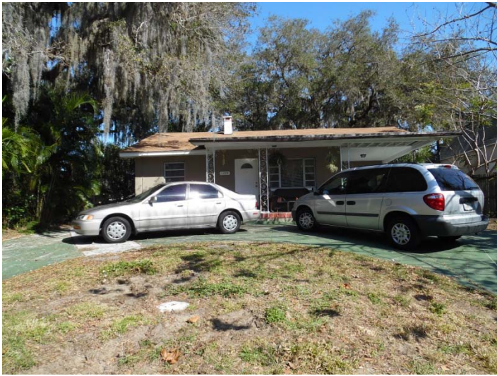
View looking north at the subject property, 1224 Sunset Point Road
