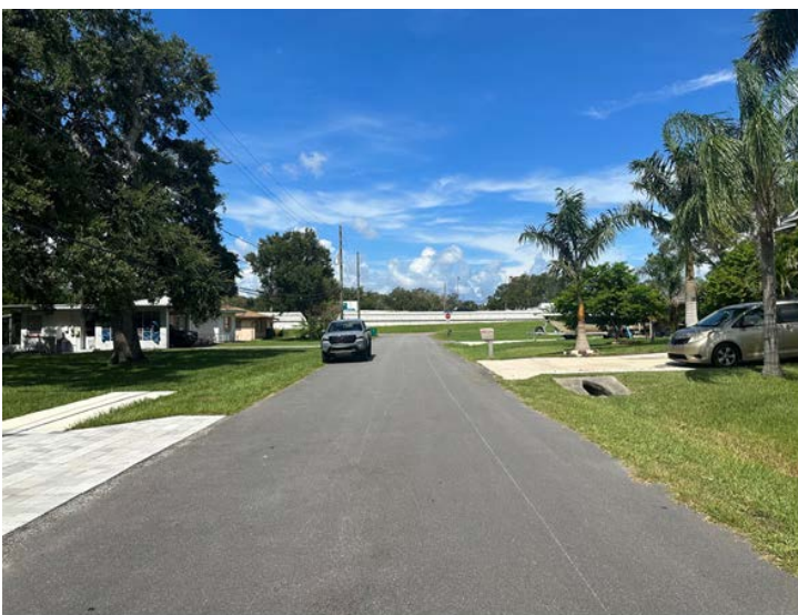
View looking westerly along Downing Street
