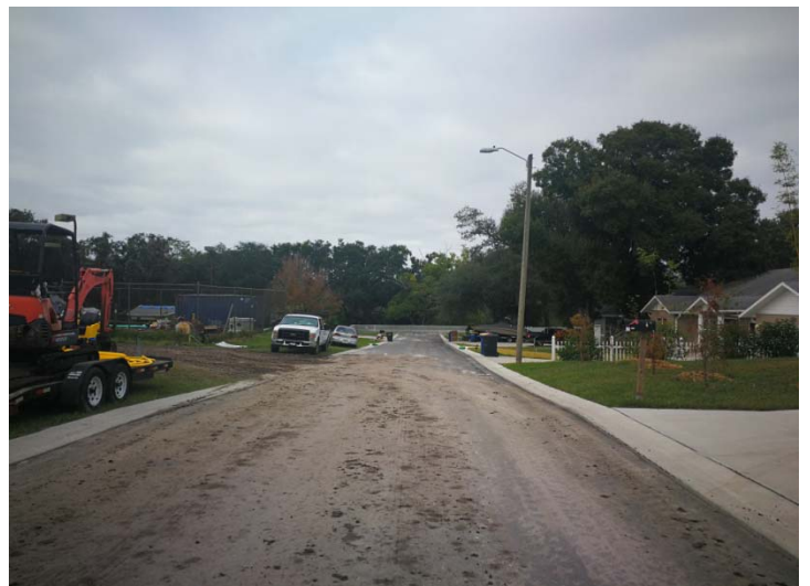
View looking westerly along Merrill Avenue
