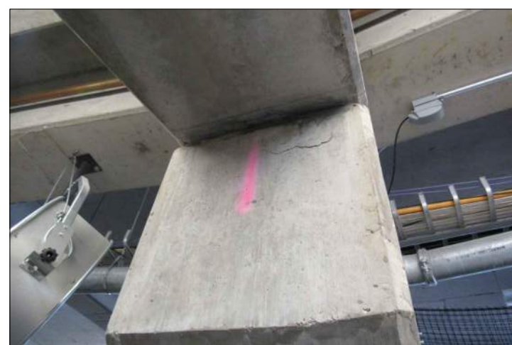
P74 CONCRETE SPALL AT C21
