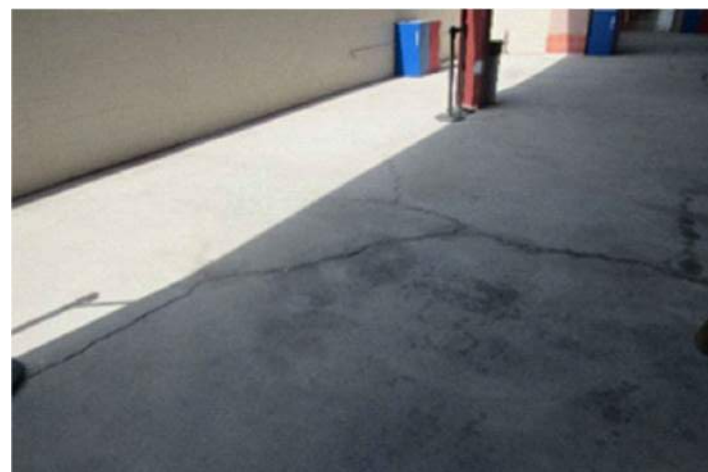
PZ36 RE-CAULK SPIDERING AT BIG SHARK, LEAK DOWN TO SOUTH GATE BELOW
