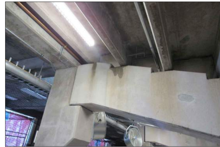
P56 LEAKS UNDERNEATH SECTION 115
