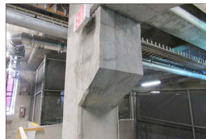
P76 CONCRETE CRACK AT C13
