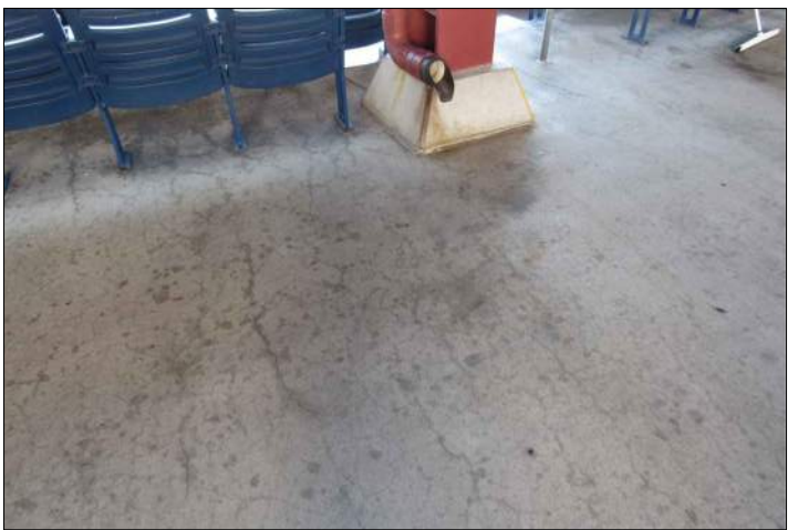
P39 CONCRETE CRACK NEAR SEATS, SECTION 111
