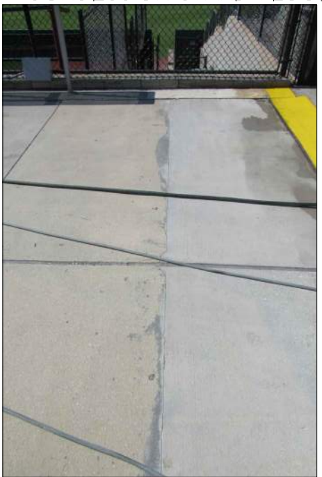
P14 CONCRETE CRACK AT TIKI 2
