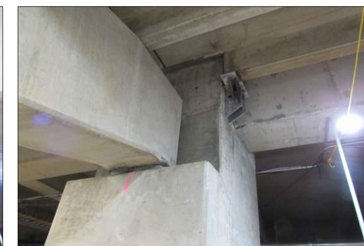
P80 CORRODED BRACKET AT C9
