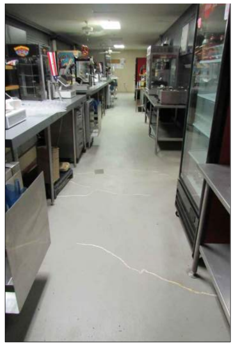
P5 LEAKS RF CONCESSION STAND/RESTROOM/RAMP INTO WAREHOUSE BELOW: RE-DO ALL CONCESSION STAND FLOORS
