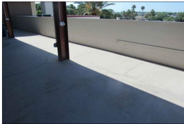
P2 CONCRETE CRACK+ LEAK FROM 3RD LEVEL BIG SHARK AREA TO THE ENTRY
