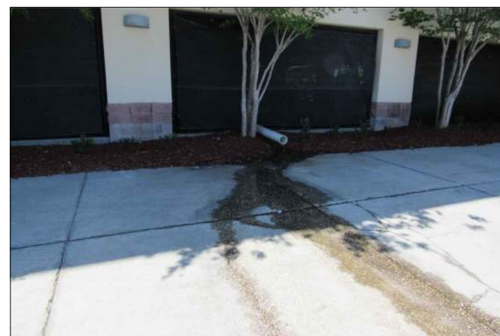
P60 EXISTING DRAIN AT SW CORNER OF STADIUM UNADDRESSED IN 2023 SURVEY; NEEDS ADDRESSING IN 2024
