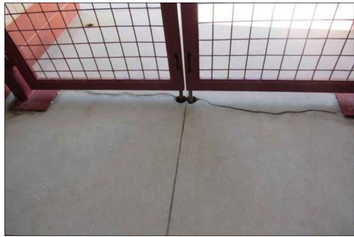
P45 GATE HOLE SLEEVES MISSING AND CONCRETE CHIPPED IN MULTIPLE LOCATIONS, WEST AND SOUTH GATES (REPLACE SLEEVE)
