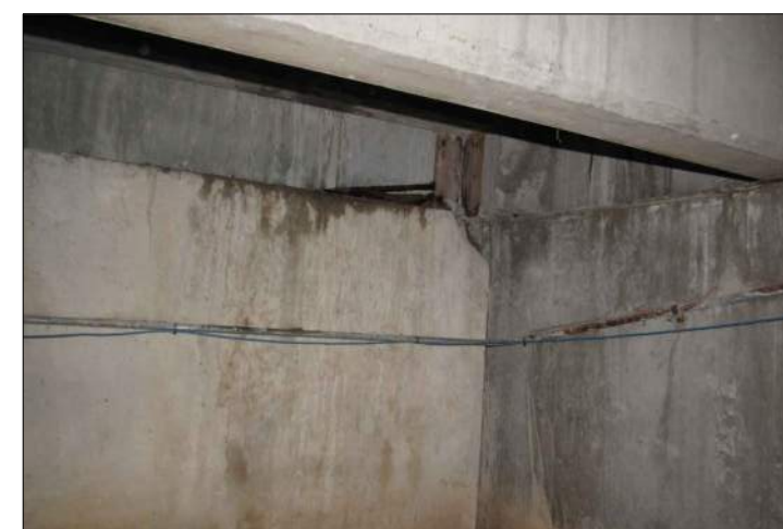
P77 LEAK AND CORRODED PAD AT A12
