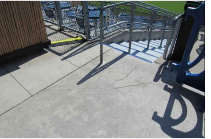
P29 CONCRETE CRACK: SECTION 120
