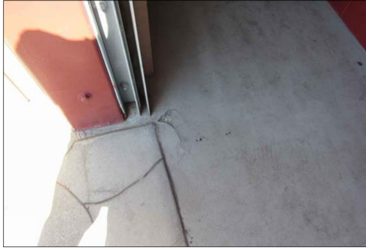
P22 CONCRETE HOLE INSIDE LF CONCESSION AT ROLL GATE (RE-DO ALL CONCESSION STAND FLOORS)
