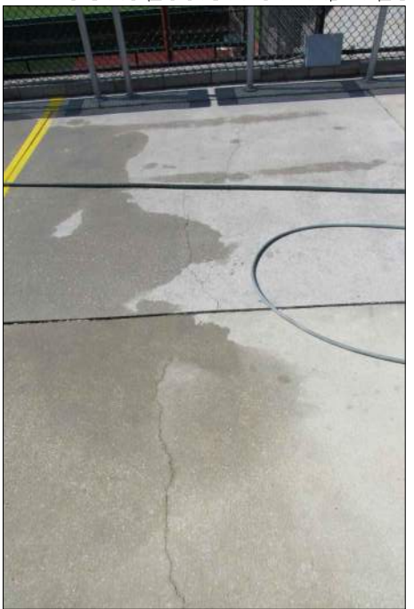
P15 CONCRETE CRACK AT TIKI 2
