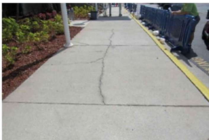
PZ50 SIDEWALK CRACKS, SOUTHSIDE (NOTE: SAFETY ISSUE)
