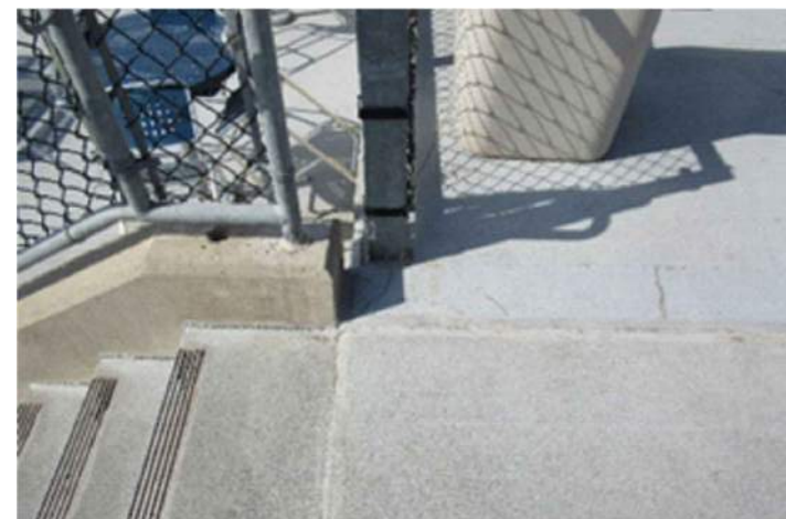
PZ13 CRACKED CONCRETE AT STAIRS OF LF PICNIC AREA
