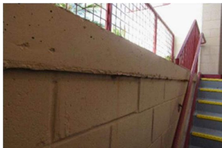
PZ35 STAIRWELL TREADS TO BE REPAINTED/RETIGHTENED & REPAIR LEAK, ELEVATOR STAIRS (ROUT/TUCK POINT OPEN JOINT)
