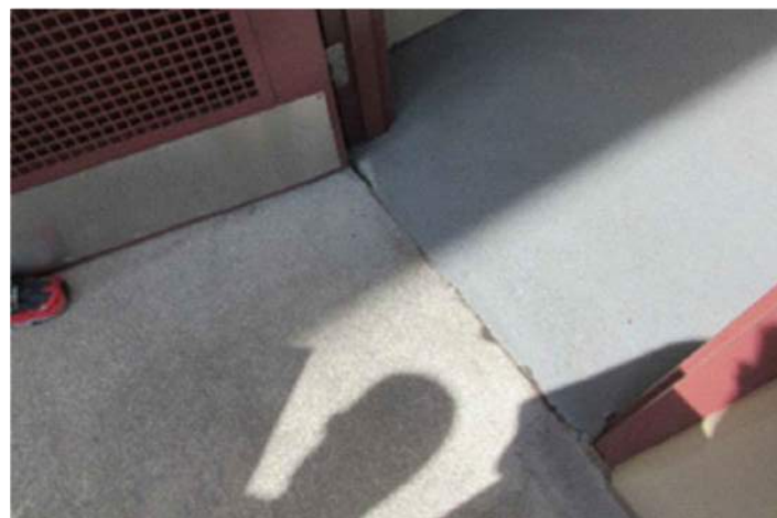
PZ11 MISSING CONCRETE AT LF MEN'S RESTROOM DOOR
