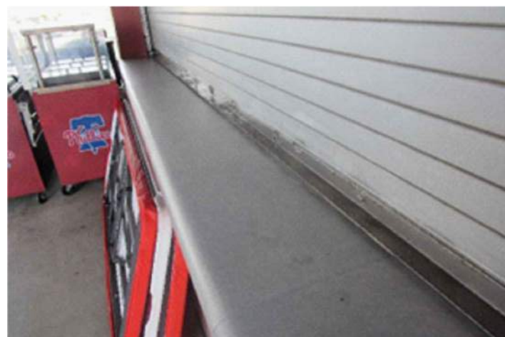
PZ37 BAY DOOR RUSTING, BIG SHARK (REPLACE DOOR SILL/SEAL)
