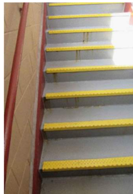
PZ34 STAIRWELL TREADS TO BE REPAINTED/RETIGHTENED & REPAIR LEAK, ELEVATOR STAIRS
