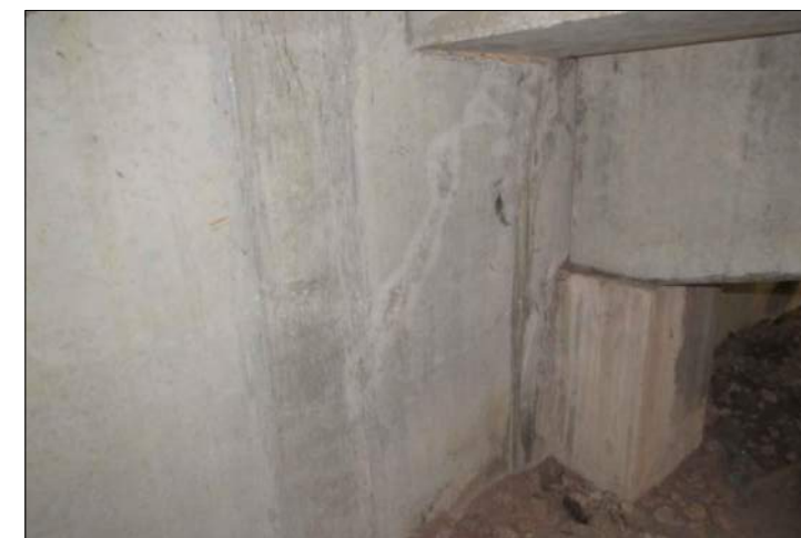
P83 CONCRETE CRACK AT A7
