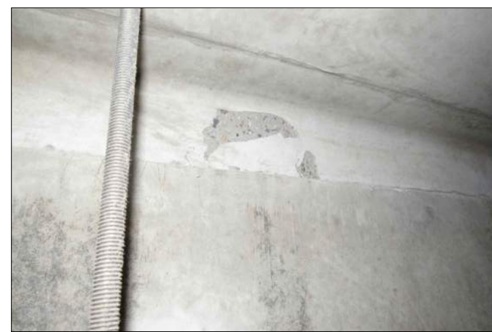
P70 CONCRETE SPALL AT C27
