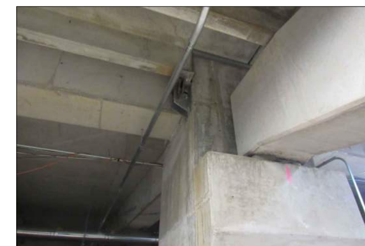
P79 CORRODED BRACKET AT C9
