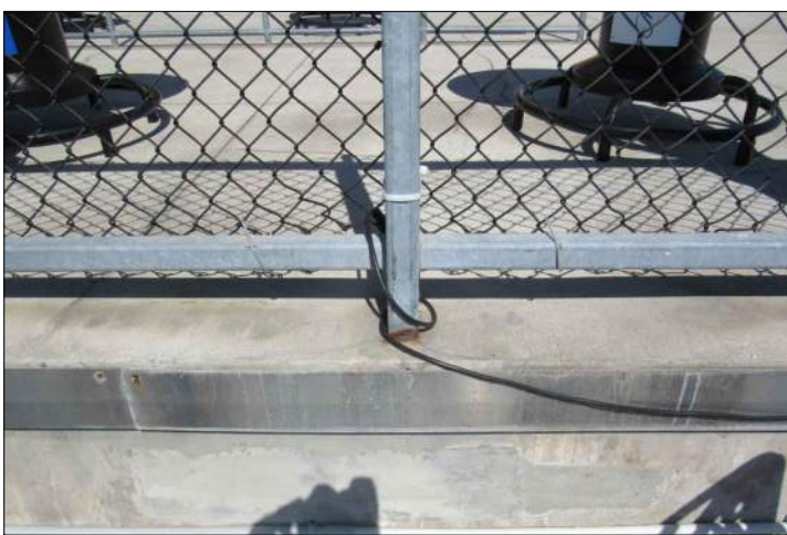
P25 CONCRETE CRACK ALONG PICNIC AREA RAILING, TOP LEVEL
