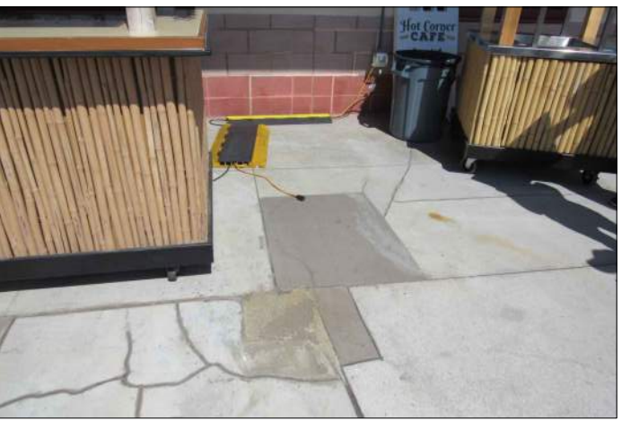
P28 CONCRETE CRACK AT OFFICE CANDLEWOOD SUITES SIGN
