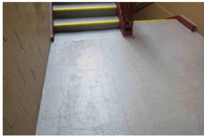
PZ20 REDO LANDINGS WITH NON-SLICK FLOORING, MIDDLE STAIRS LANDING
