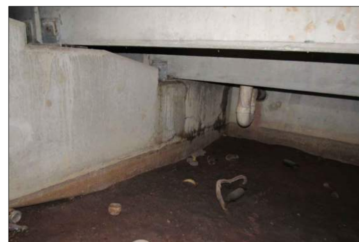
P75 RAINWATER LEAK AT C20
