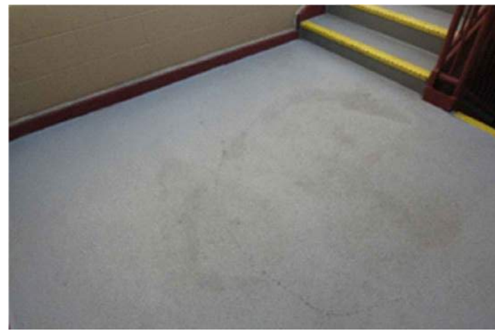
PZ21 REDO LANDINGS WITH NON-SLICK FLOORING, MIDDLE STAIRS LANDING
