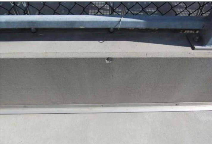
P19 EXPOSED REBAR AT TIKI TIERS WALLS, FIRST AND SECOND LEVEL
