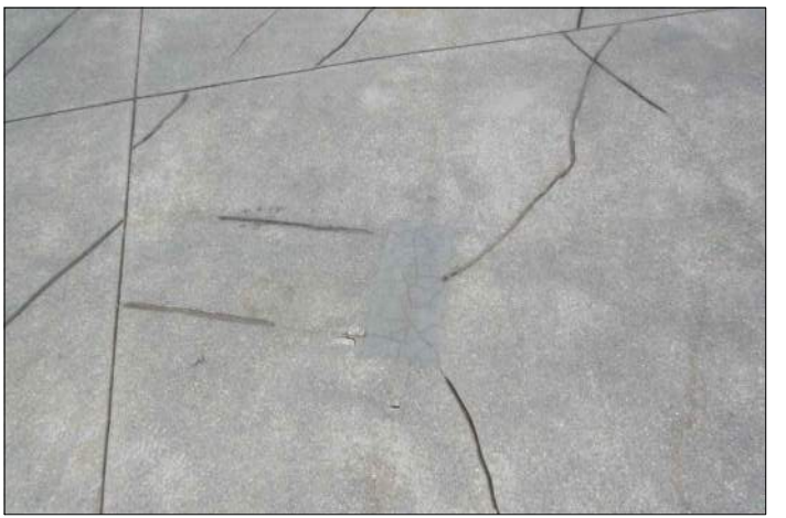
P27 EXPOSE REBAR IN KID ZONE
