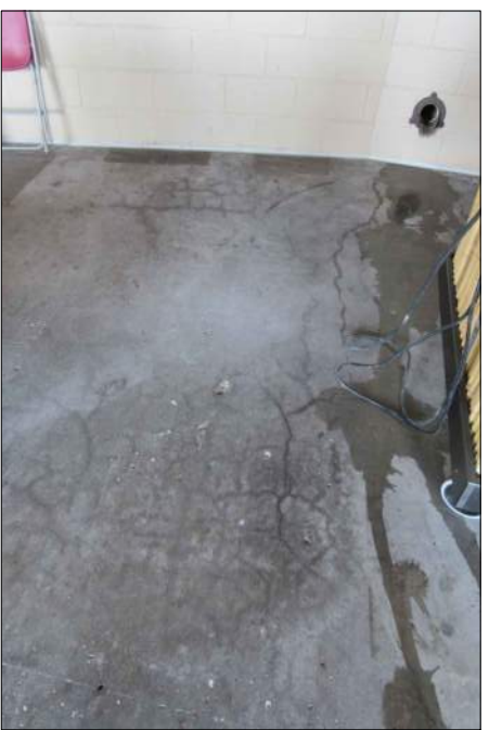
P38 CONCRETE CRACK & CRAZING AT SHERATON SIGN, SECTION 112
