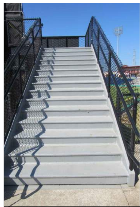
6 P12: BETTER'S EYE STAIRS TO BE RE-DONE 1: POWER WASH 2: REMOVE ALL LOOSE MATERIAL. 3: RE-COAT WITH SIKALASTIC 350. 4: SEE SPECIFICATIONS.
