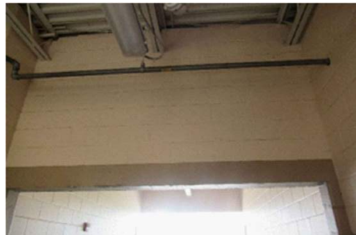
PZ42 RAMP DOORWAY REMOVAL OR EXPANSION (RAISE CIP CONCRETE LINTEL BY 16")
