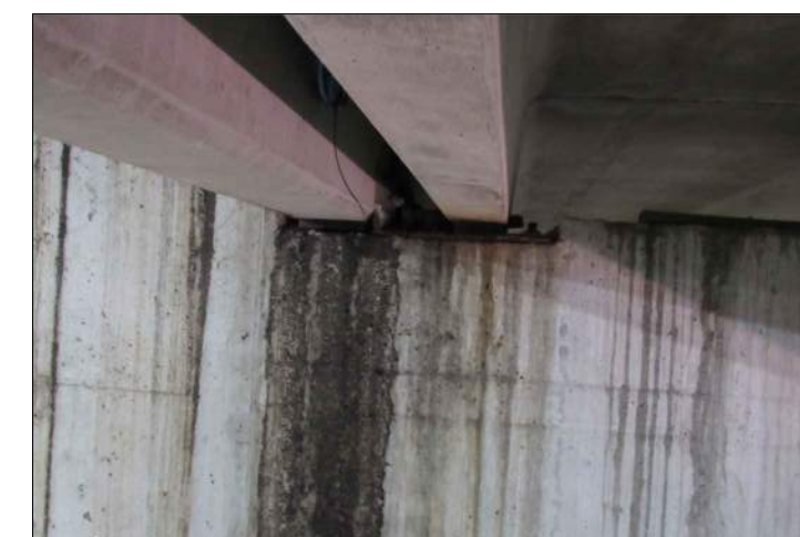
P86 LEAK AND CORROSION AT BATTING CAGE
