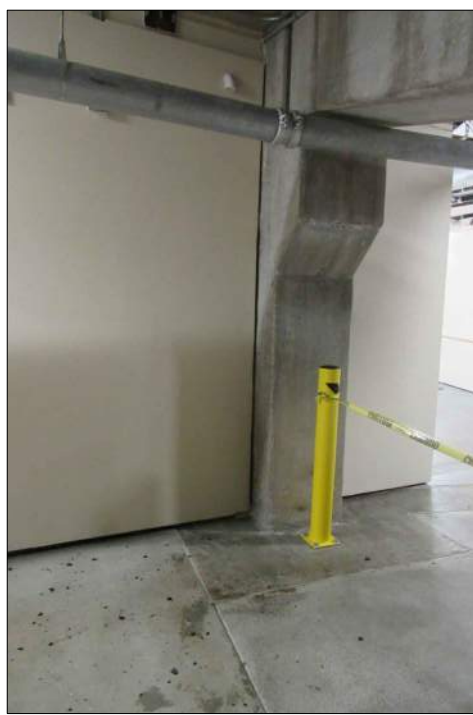
P53 LEAKS UNDERNEATH SECTION 108
