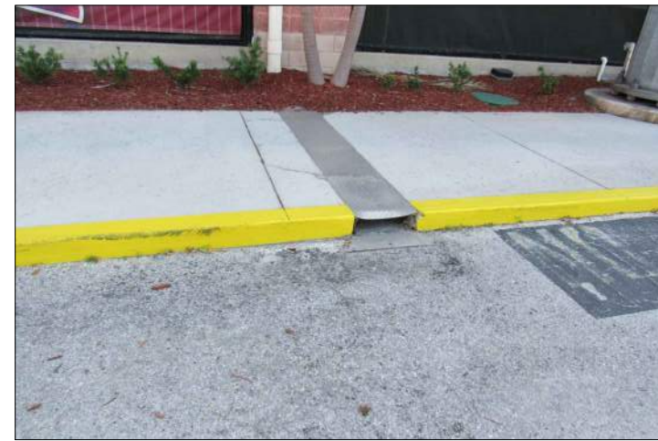
P57 REPLACE/REPAIR REST OF DRAIN BOXES ALONG EXTERIOR
