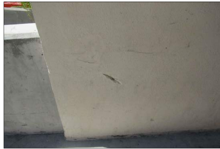
P48 EFIS REPAIRS REQUIRED AT RAMP AND OTHER LOCATIONS THROUGHOUT FACILITY
