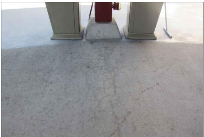
P41 SPIDERING CONCRETE CRACK THROUGHOUT MAIN CONCOURSE
