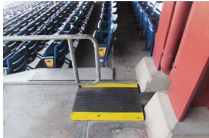
PZ23 EXTEND RAILING AT SECTION 108 (TOP/HANDICAP AREA) TO BLOCK SECTION 107 (NOTE: SAFETY ISSUE)
