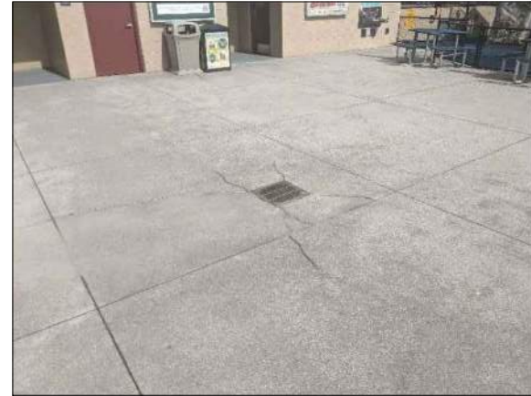
PX5 DRAIN ABOVE OFFICE LEAK
