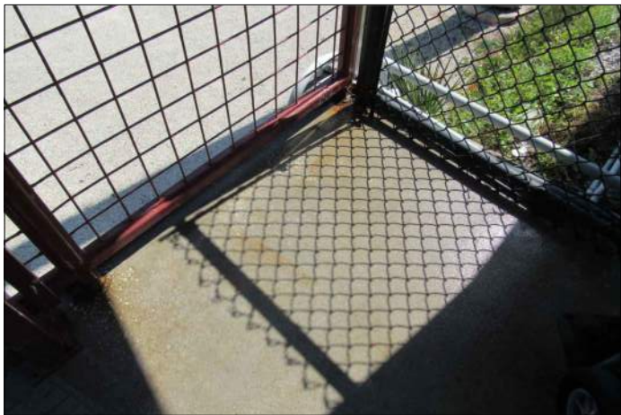
P16 RUSTING AT RAILING ALONG TIKI BAR AT TIKI 2 AND STAGE
