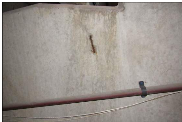
P68 EXPOSE REBAR AT C28
