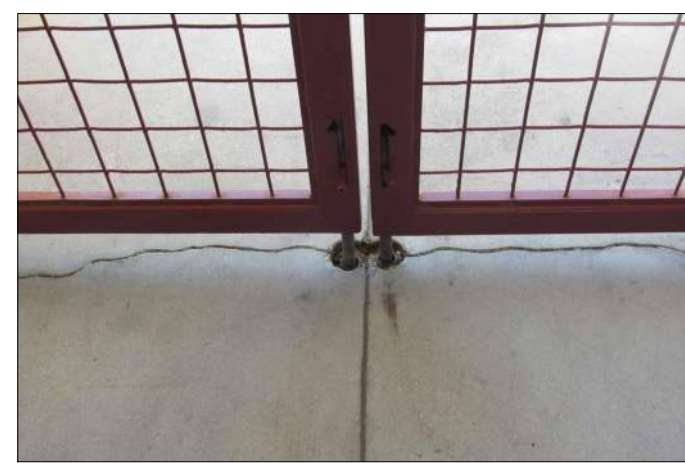
1 P46: GATE SLEEVES MISSING AT ENTRY GATES 1: EXCAVATE THE REMNANTS OF THE EXISTING SLEEVES. 2: INSTALL NEW HDG SLEEVES TO MATCH EXISTING. 3: REPAIR CONCRETE WITH A REPAIR MORTAR.
