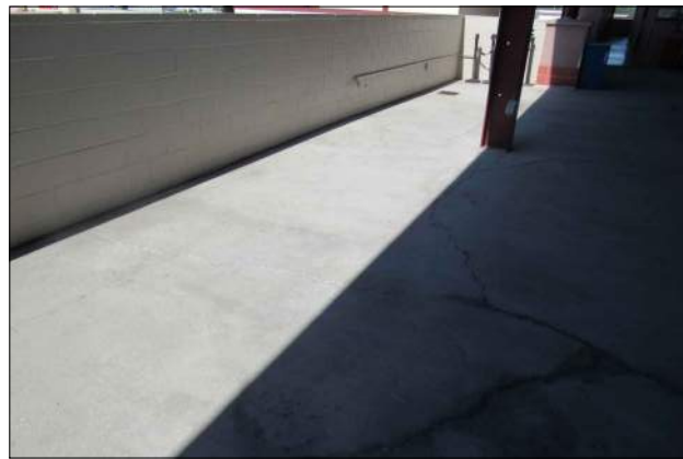
P1 CONCRETE CRACK+ LEAK FROM 3RD LEVEL BIG SHARK AREA TO THE ENTRY GATE
