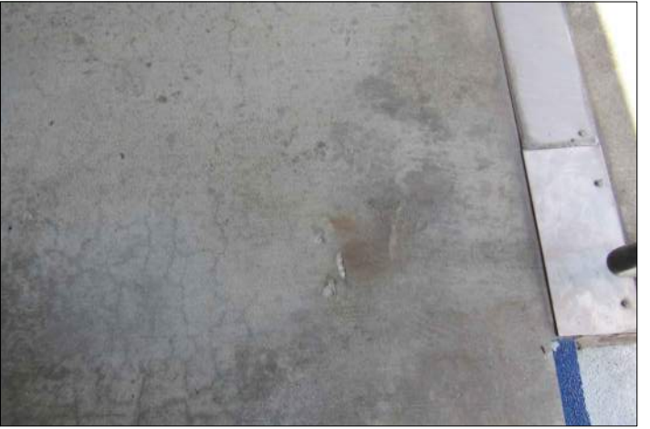
P33 CHIPPED CONCRETE AT HANDICAP AREA, SECTION 114
