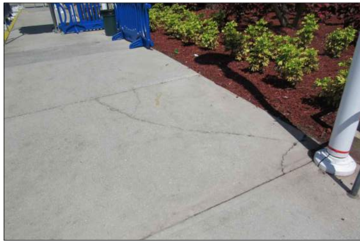
P51 CONCRETE CRACK AT TOP OF SUITES RAMP
