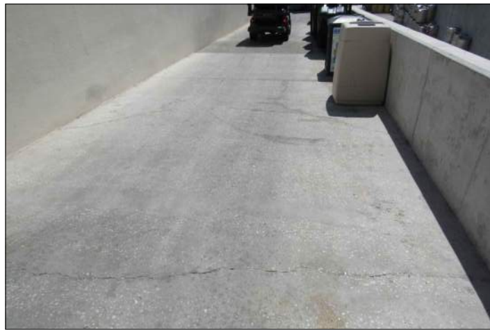
P47 CONCRETE CRACK ALONG RAMP
