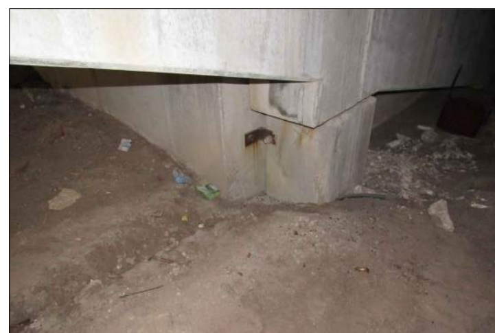
P82 CORRODED BRACKET AT B8
