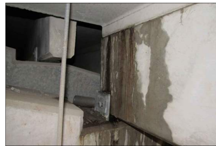
P69 LEAK AT C27
