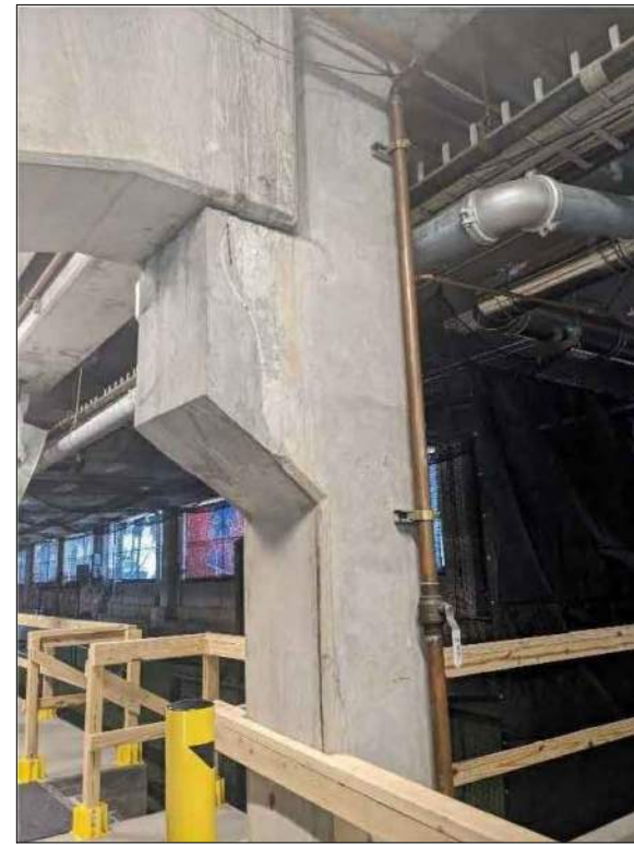
PX12 CONCRETE CRACK, C14
