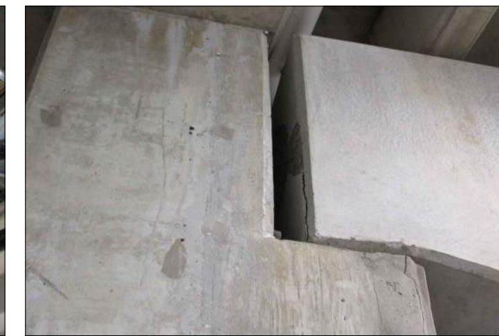
P73 CONCRETE CRACK AT C23
