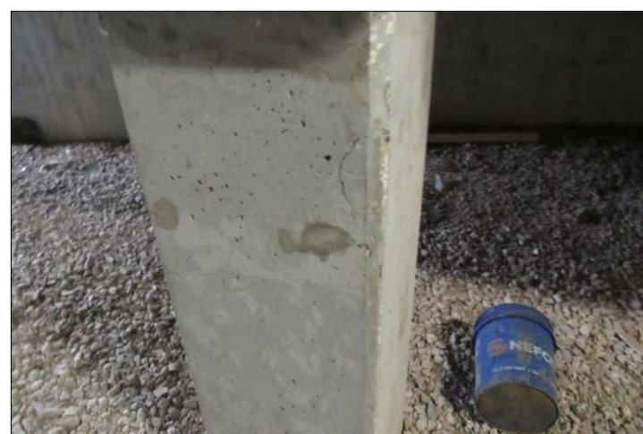
P84 CONCRETE SPALL AT C5.5
