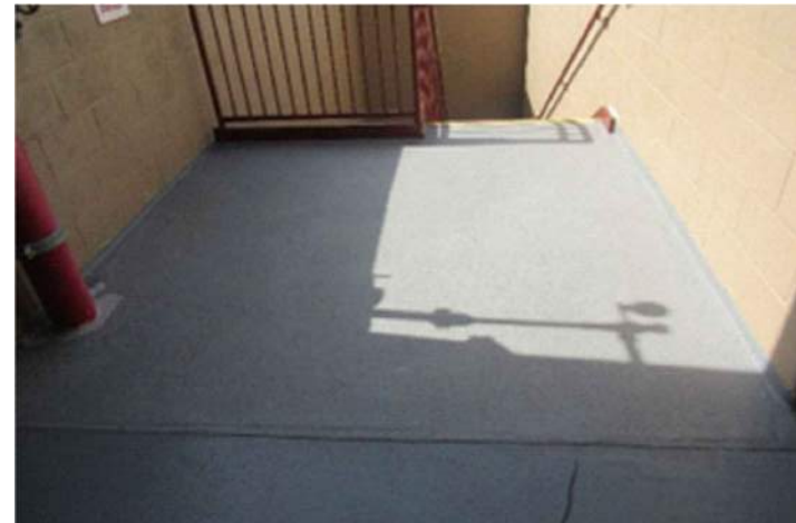
PZ22 REDO LANDINGS WITH NON-SLICK FLOORING, MIDDLE STAIRS LANDING
