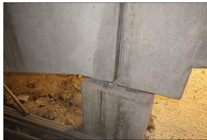
P66 CONCRETE CRACK AT C29
