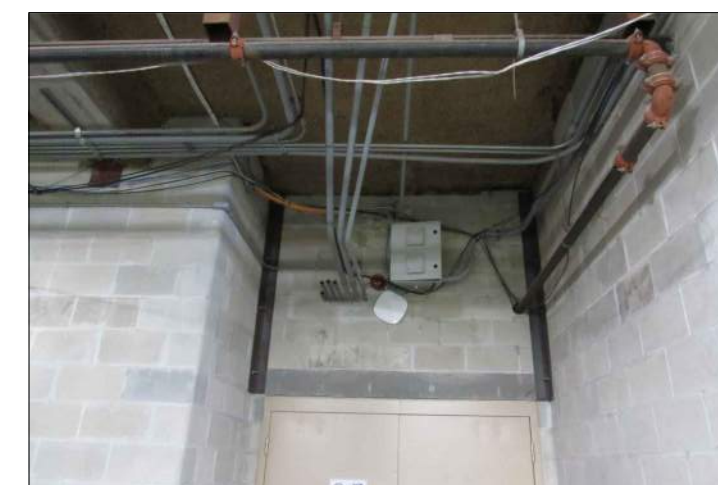
P87 RUSTED BRACKETS AT BATTING CAGE
