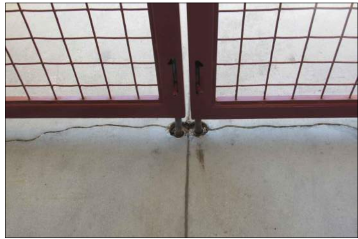
P46 GATE HOLE SLEEVES MISSING AND CONCRETE CHIPPED IN MULTIPLE LOCATIONS, WEST AND SOUTH GATES (MAINTAINED SLEEVES, PICTURED)
