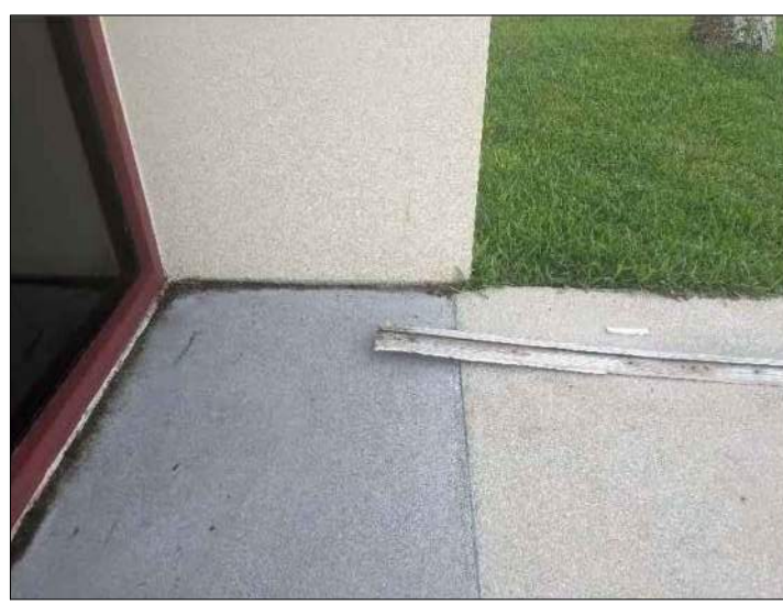
PX2 HALF-INCH RECESS AT OFFICE, GROUND LEVEL
