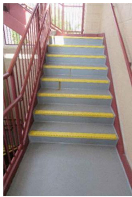
PZ18 STAIRWELL TREADS TO BE REPAINTED/RETIGHTENED, ELEVATOR STAIRS IN ARCH
