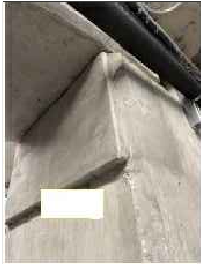
PX23 C23 (SEVERE CRACKING)
