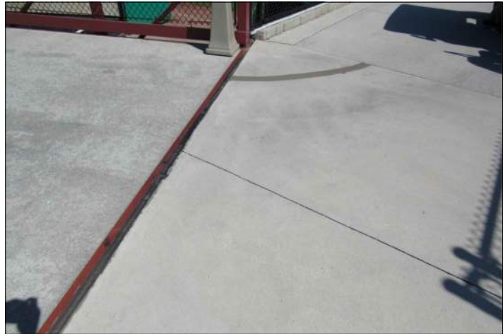
P11 CONCRETE CRACK AT BRIDGE
