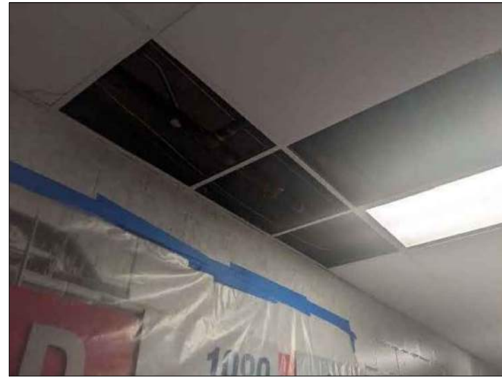
PX4 LEAK IN CEILING, OFFICE HALFWAY AT HALL LEVEL
