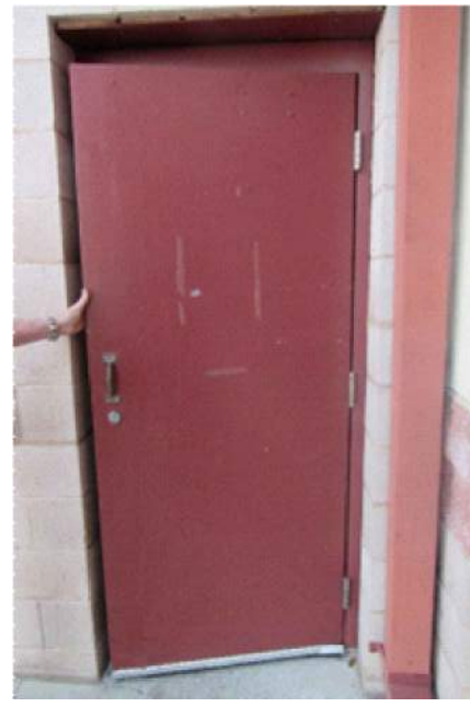
PZ59 REPLACE BOTTOM OF WEST STAIRWELL DOOR (BENT)
