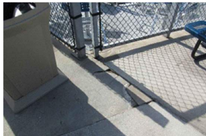
PZ12 CONCRETE REPAIR & MISSING CAULKING AT CORNER OF LF PICNIC
