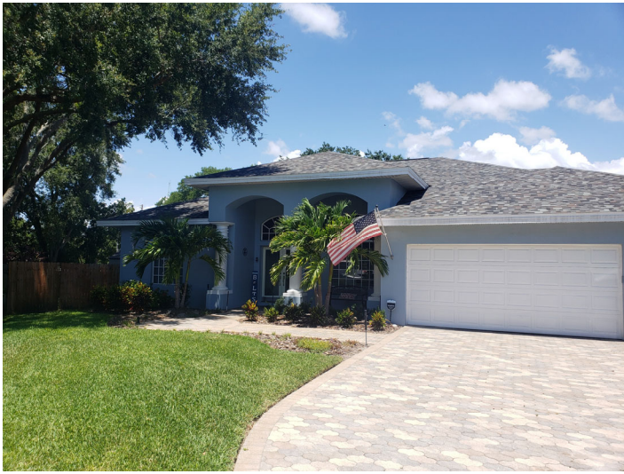
View looking northeast at subject property 3467 Sweetwater Trail
