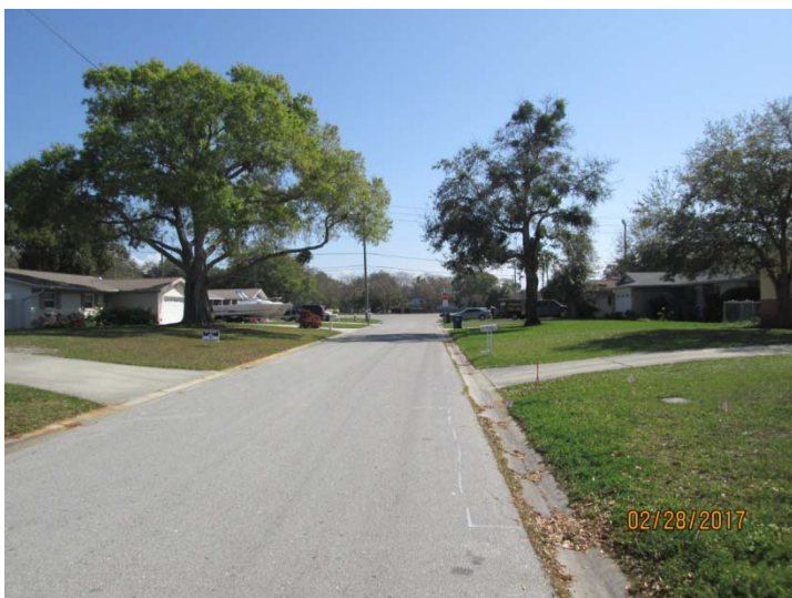
View looking easterly along Hoyt Avenue
