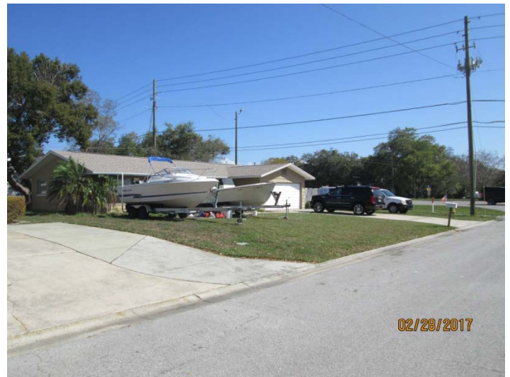
East of the subject property
