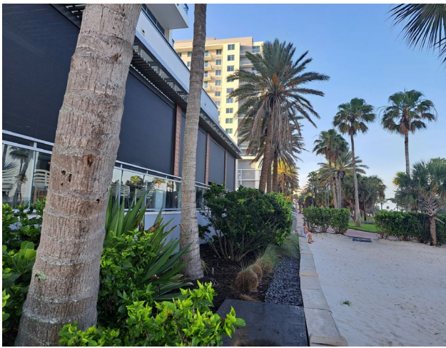
Facing southwest at the subject property along the west façade of the Wyndham Grand.
